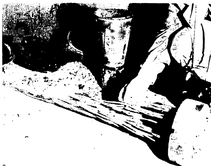
Fig. 6: Rupture of the tendon in the form of a bevel near its anchoring head.
