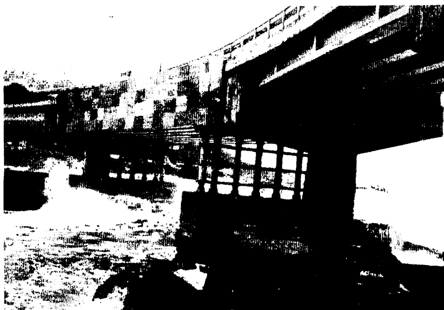
Fig. 16: Construction of additional supports in Kuretsubo Bridge [1]
