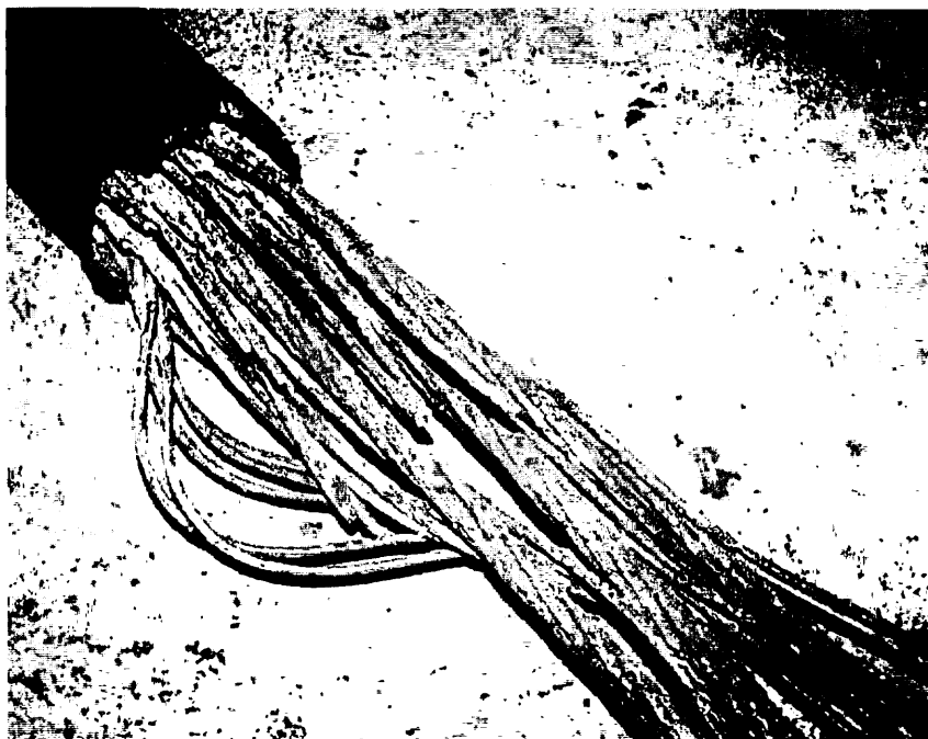
Fig. 8: Corrosion and broken wires in the failure zone.
