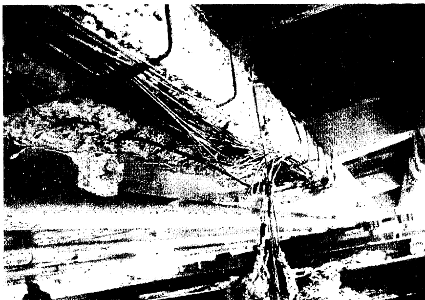
Fig. 17: Breaking of prestressing tendons in Kuretsubo Bridge [1]
