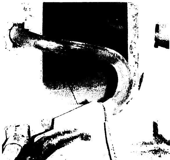
Fig. 5: Large lateral deformations of the broken tendon near a crossbeam.
