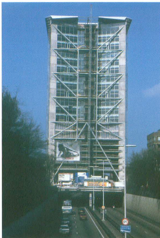
Fig. 1-7: Precast concrete, cast insitu concrete and steelwork in the VNO Building, Netherlands. (Courtesy of Corsmit Consulting Engineers, Netherlands)
