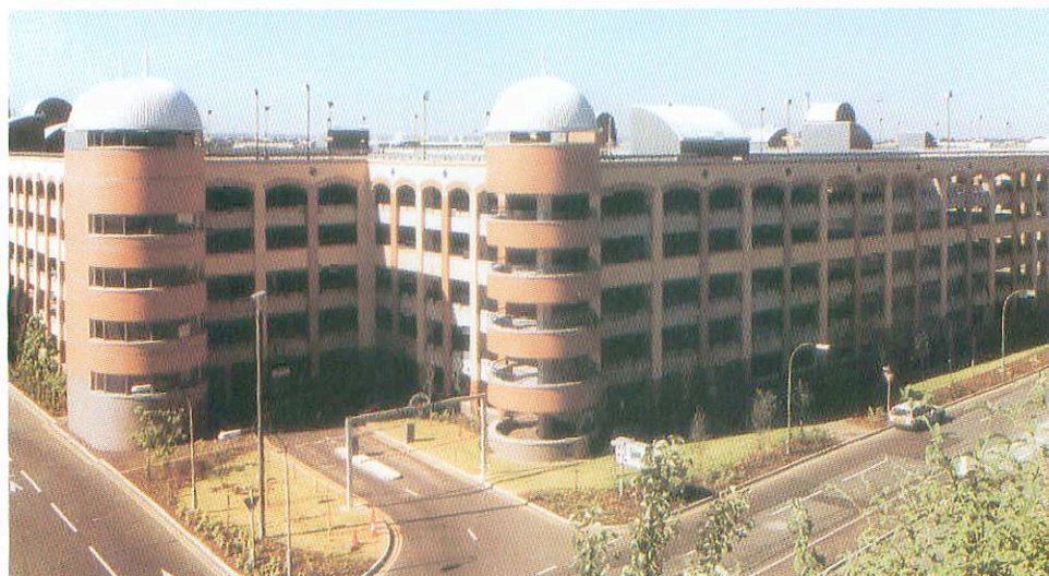
Fig. 2-14: Precast and cast insitu concrete combined to construct 3000 parking spaces in 8 months. (Courtesy of Reinforced Concrete Council, UK)
