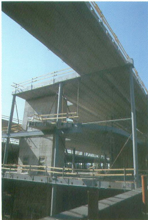
Figs 3-6 (left) and 3-7 (right): Concrete filled tubular steel columns and shallow prefabricated steel box beams support precast hollow core floor slabs. 'The Big Apple', Helsinki.
