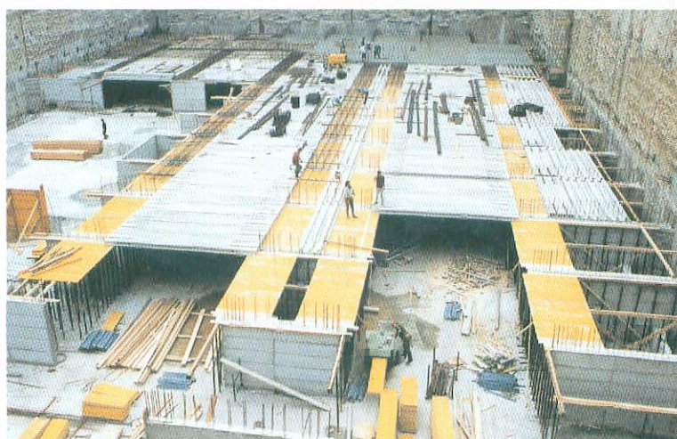
Fig. 2-4: Wide insitu concrete beams supporting precast concrete hollow core floors at an underground car park, Parma, Italy. (Courtesy of Gruppo Centro Nord, Italy)
