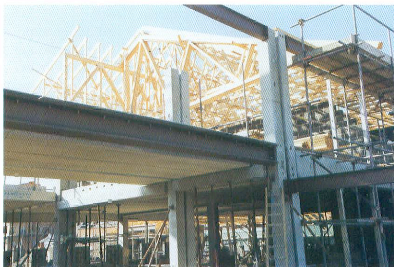
Fig. 1-6. Mixed construction using different building materials was used – cast insitu and precast concrete, steelwork, timber, masonry. Offices and Car Park, Nottingham, UK.
