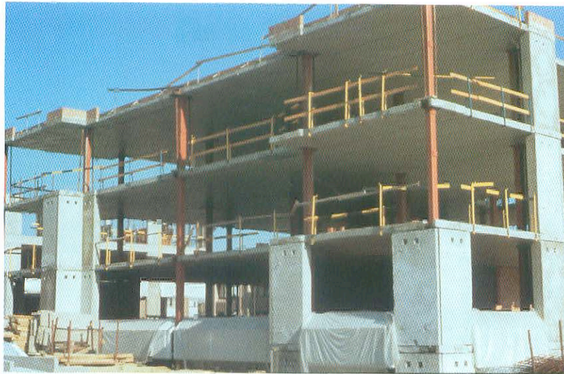
Fig. 1-10: Steel columns in a concrete lift slab braced by precast walls.
