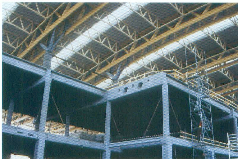
Fig. 4-6: Interior view during construction of precast frame and timber rafters at Oslo International Airport. (Courtesy of Spenncon, Norway)
