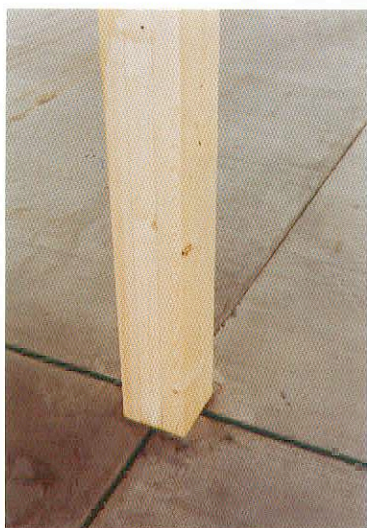
Fig. 4-8: Glue laminated timber beams and columns support precast flooring in a warehouse (Courtesy of Strängbetong, Sweden)
