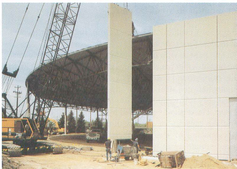
Fig. 3-30: Vertical precast sandwich panels used in steel frame warehouses, stadia etc. (Courtesy of PCI, USA)
