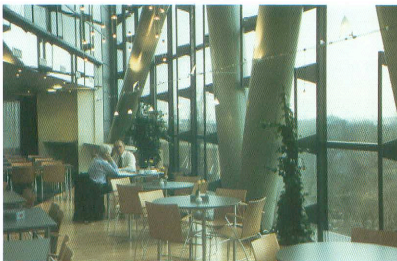
Fig. 1-8: Interior view at VNO showing tubular steel bracing and precast concrete floors (now screeded finish). (Courtesy of Corsmit Consulting Engineers, Netherlands)
