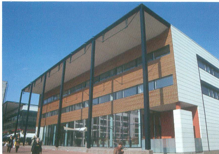
Fig. 1-11: Precast concrete, steel, timber and glazing all feature in this building in Helsinki, Finland.
