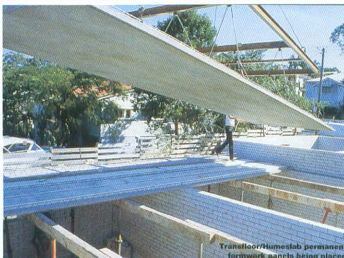
Fig. 5-3: Permanent precast concrete formwork ('half-slab') floor units spans across an intermediate brickwork wall (Courtesy of Cement & Concrete Association of Australia)
