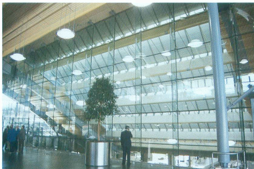
Fig. 4-7: Structural timber and glazing systems supported from the precast frame at Oslo International Airport.
