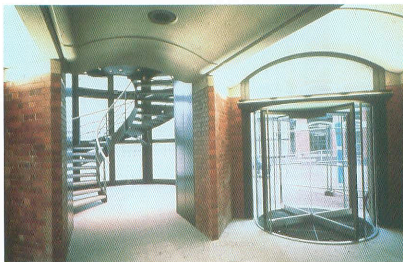
Fig. 5-9: Interior view of prefabricated brick pillars and exposed precast floor units at Inland Revenue, Nottingham, UK. (Courtesy of Brick Development Association, UK)
