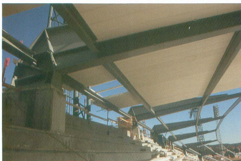
Fig. 3-28: Steel roof beams cantilevered from the top of precast concrete columns
