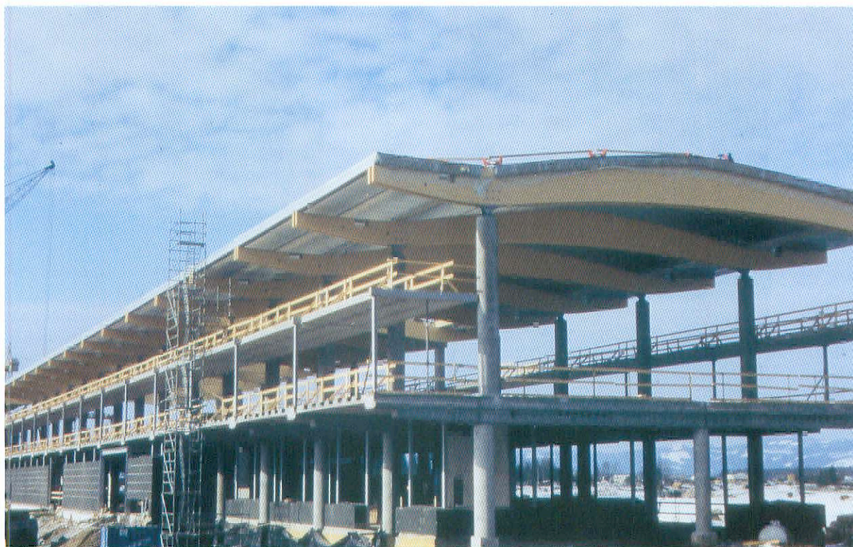
Fig. 1-1: Mixed construction using precast concrete and timber, both indigenous materials to the local construction industry in Norway (Courtesy Spenncon, Norway)
