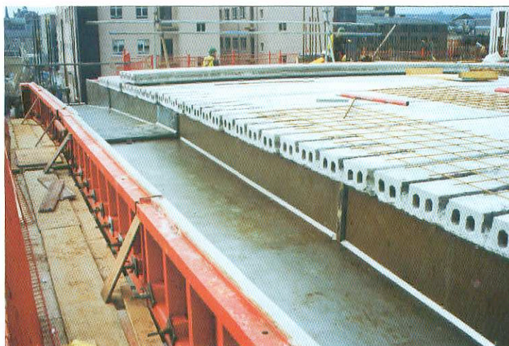
Fig. 2-8: Precast U-shape or shell beams awaiting post tensioning. (Courtesy of Concrete Society, UK)
