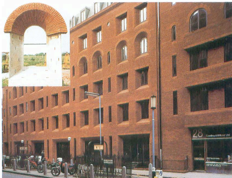
Fig. 5-6: Structural precast concrete spandrel beams with integrated brickwork façade (Courtesy of Trent Concrete Ltd., UK)
