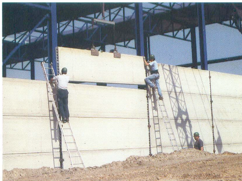
Fig. 3-31: Horizontal hollow core wall panels used in a steel frame warehouse (Courtesy of Echo, Belgium)
