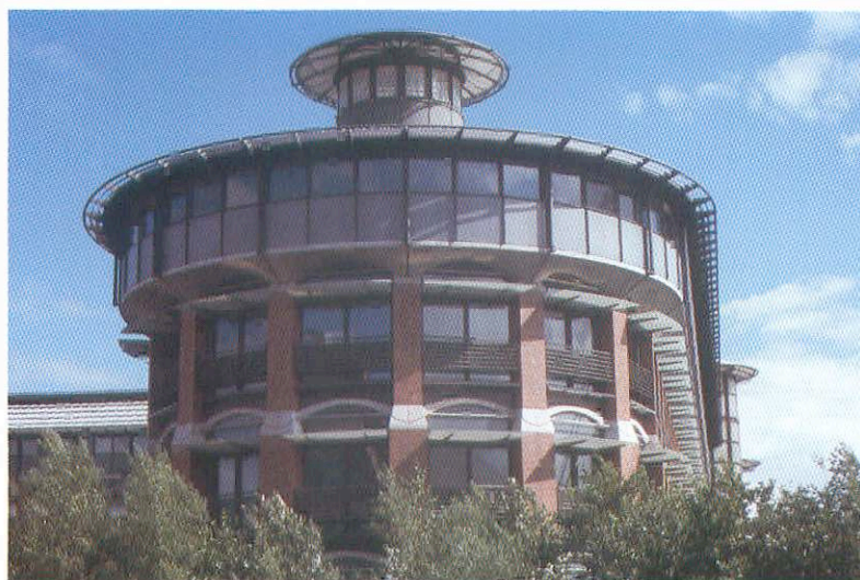
Fig. 5-8: Prefabricated brickwork pillars support precast concrete floors and steel roof at the rotunda, Inland Revenue, Nottingham, UK.
