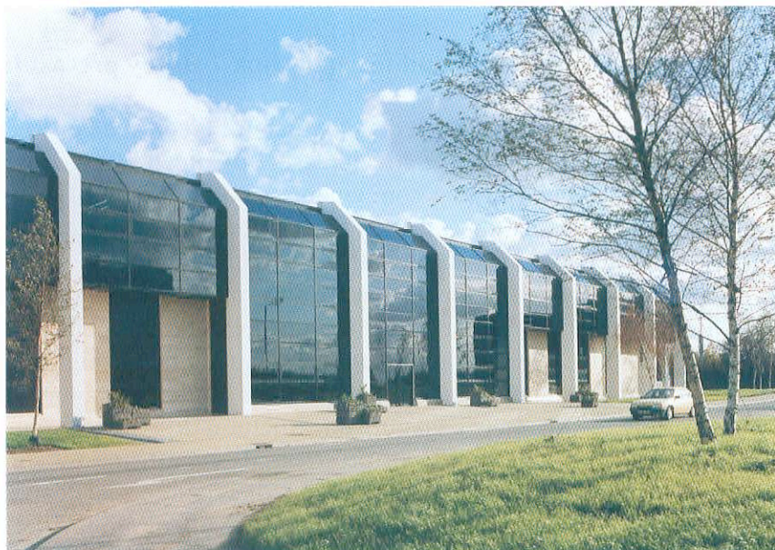
Fig. 1-5: Architectural / structural precast columns in white concrete support steel roof lattices. (Courtesy of British Cement Association, UK)
