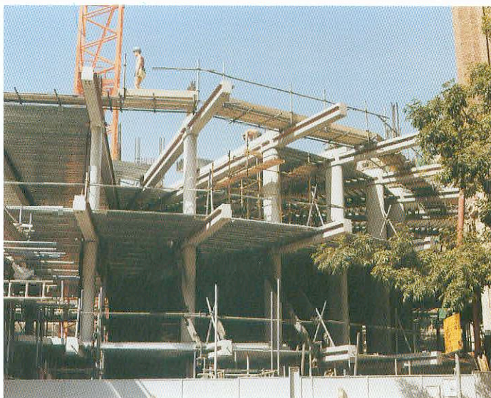
Fig. 3-15: Profiled metal decking supported on cantilevered precast beams. Bracken House, London (Courtesy of Trent Concrete Ltd. UK)
