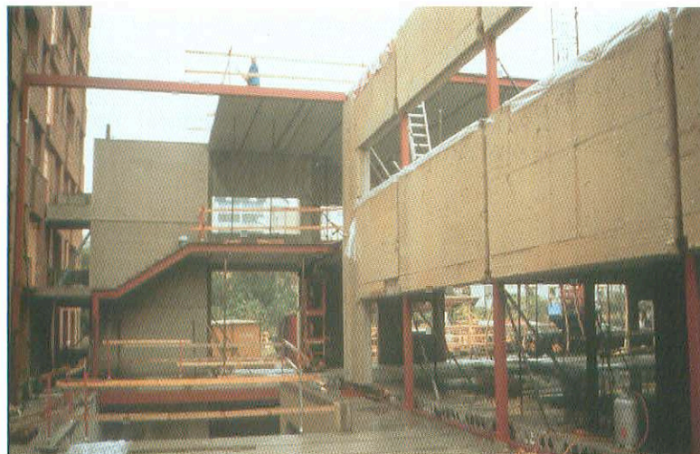
Fig. 3-19: Insulated precast concrete spandrel units and precast shear cores in a steel frame near Stockholm (Courtesy of Strängbetong, Sweden)
