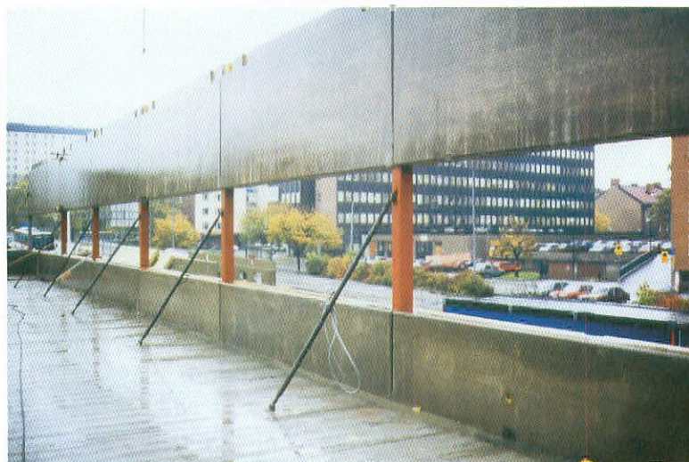
Fig. 3-18: Precast concrete spandrels and hollow core flooring in a steel frame near Stockholm, Sweden. (Courtesy of Strängbetong, Sweden)
