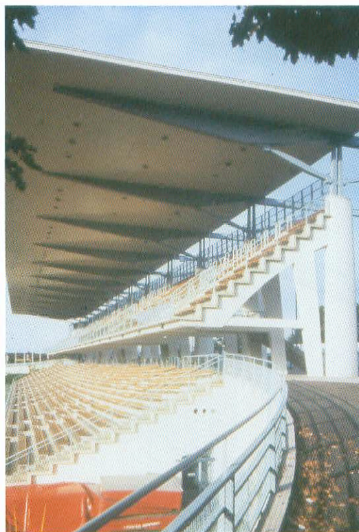
Fig. 3-27: Balanced steel beams forms the roof on top of a precast grandstand structure (Courtesy of Parma Betonila, Finland)
