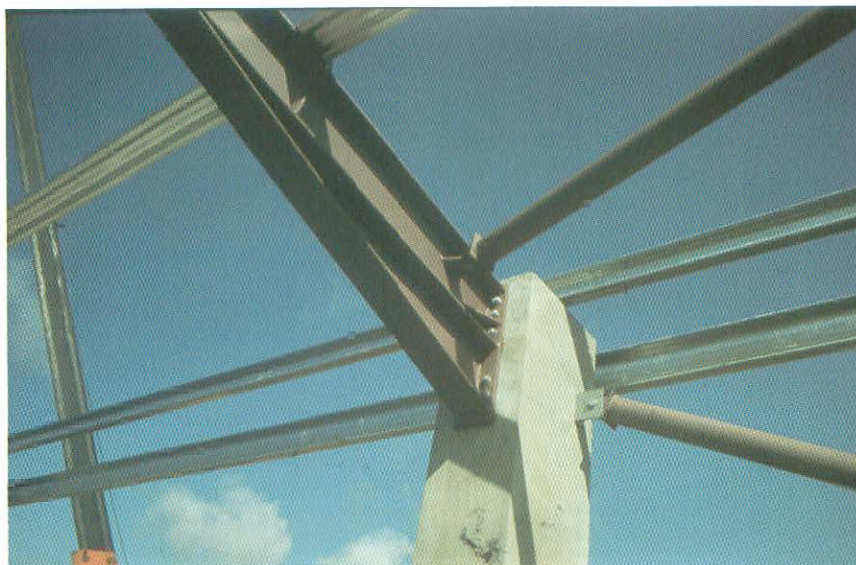
Fig. 3-21: Structural steelwork to precast concrete connection details
