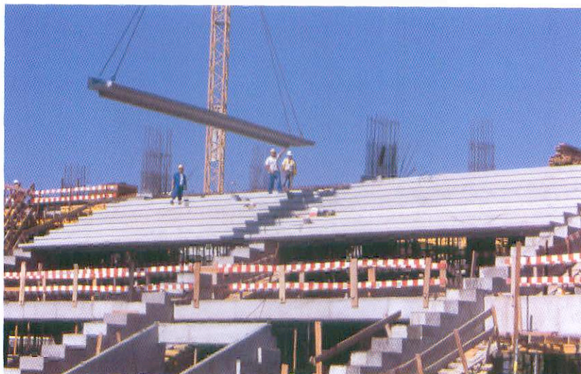
Fig. 2-11: Precast terracing units being placed onto cast insitu raker beams at Sporting Lisbon FC, Portugal, soccer ground.
