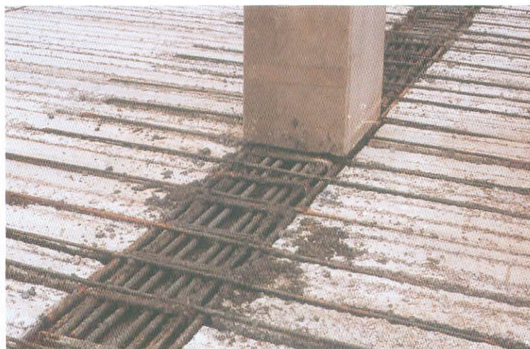
Fig. 2-3: Completion of precast – cast insitu floor. Offices, Turin, Italy. (Courtesy of Gruppo Centro Nord, Italy)
