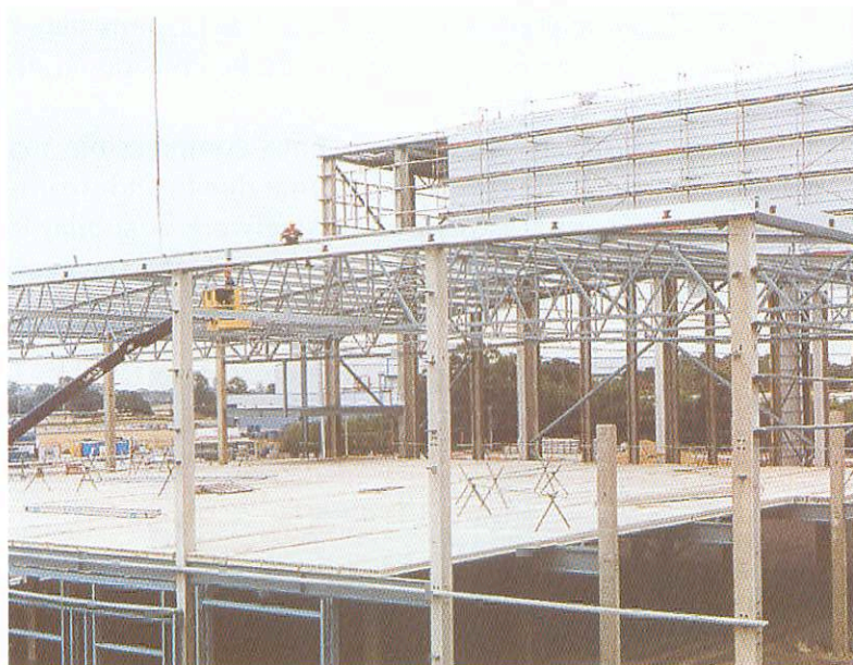
Fig. 3-25: Steel trusses atop 25 m high prestressed precast concrete columns (Court. Composite Structures, UK)
