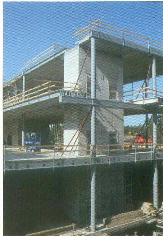
Figs 3-6 (left) and 3-7 (right): Concrete filled tubular steel columns and shallow prefabricated steel box beams support precast hollow core floor slabs. 'The Big Apple', Helsinki.
