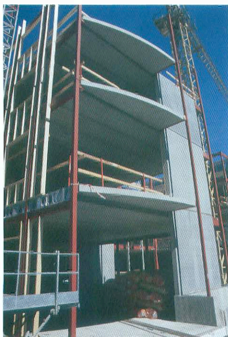
Fig. 1-2: Mixed precast concrete and structural steelwork
