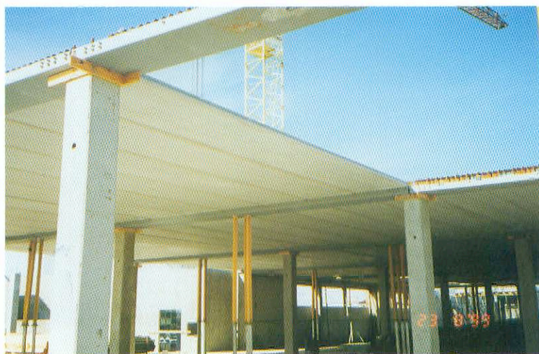
Fig. 3-11: A steel shell beam and a rebar cage supports hollow core floor units. (Courtesy of Addtek International Ltd, Finland)
