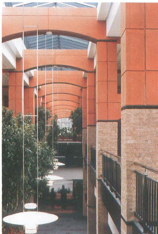
Fig. 5-7: Prefabricated brickwork pillars support architectural precast concrete arches (Courtesy of Trent Concrete Ltd. UK)
