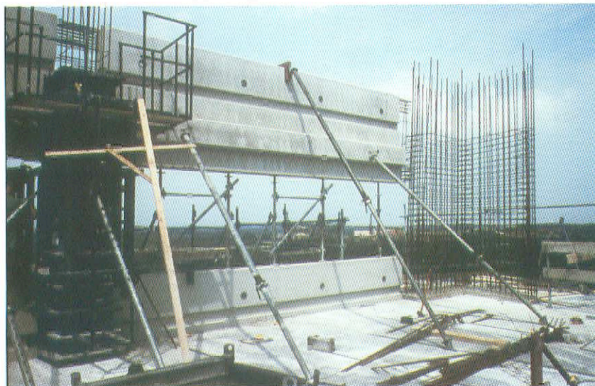
Fig. 2-19: Precast concrete spandrels attached to cast insitu columns at VNO Building, Netherlands. (Courtesy of Corsmit Consulting Engineers, Netherlands)
