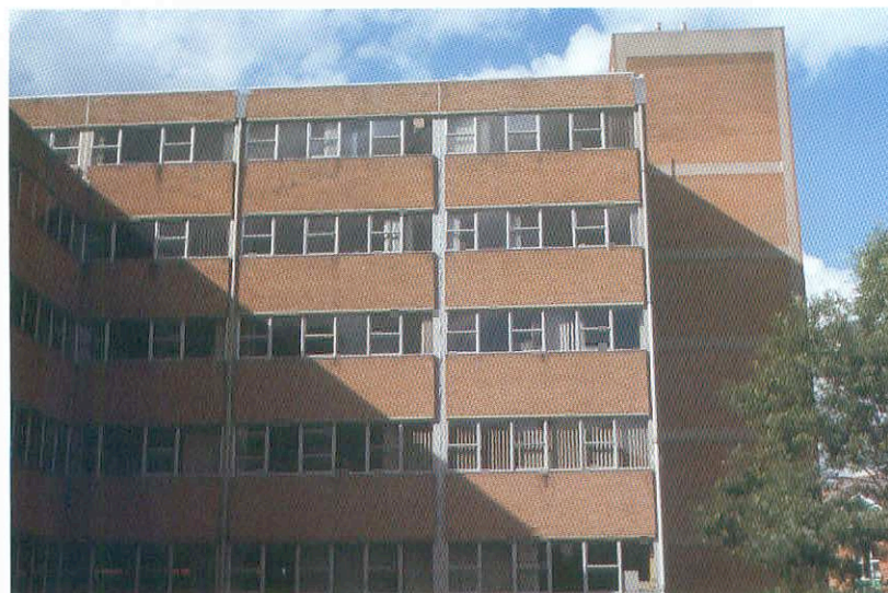
Fig. 5-10: Infill brick walls used to stabilise pin-jointed precast concrete frames
