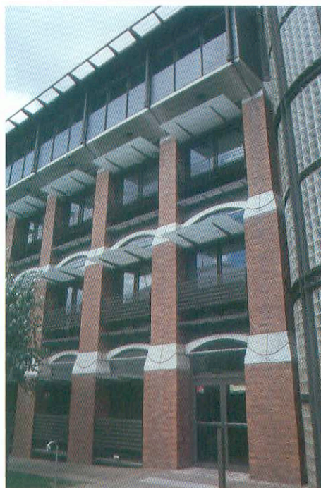
Fig. 1-3: Precast concrete floors and brick pillars form both the structural elements and the architectural façade.
