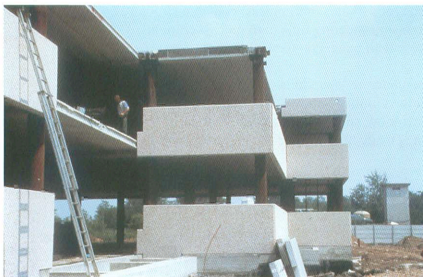
Fig. 3-20: Exposed finish panels on a steel frame
