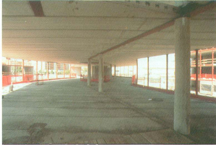
Fig. 3-5: Long spans and a flush soffit are a feature of placing precast floor units onto the bottom flanges of steel beams. (Courtesy of Strängbetong, Sweden)
