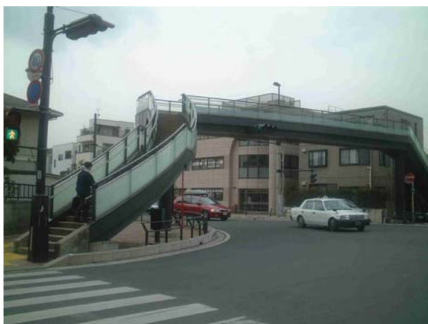
Fig 3.4 Typical pedestrian footbridge in Japan
