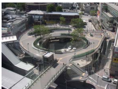
Fig. 2.2 Pedestrian deck at Station Plaza
