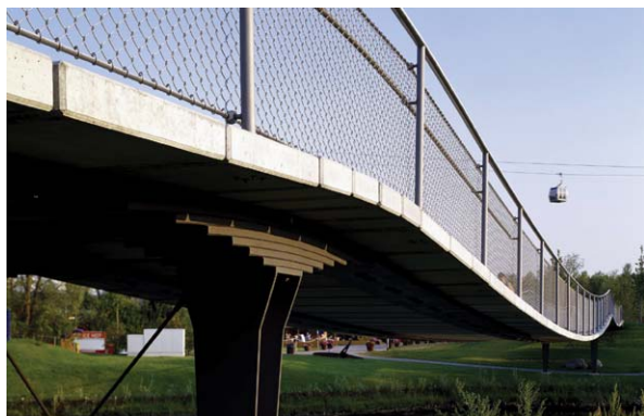
Fig. 5.20 Heavy deck surfacing and chain-link railing at the Nordbücke in Rostock, Germany
