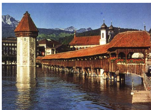
Fig. II.1 Chapel Bridge in Lucerne, Switzerland
