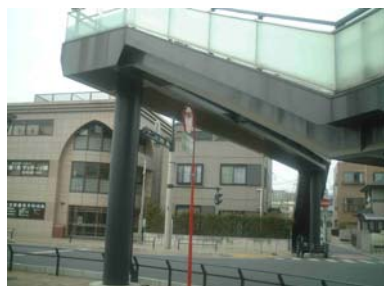
Fig. 2.1 Board screens on a footbridge in Japan
