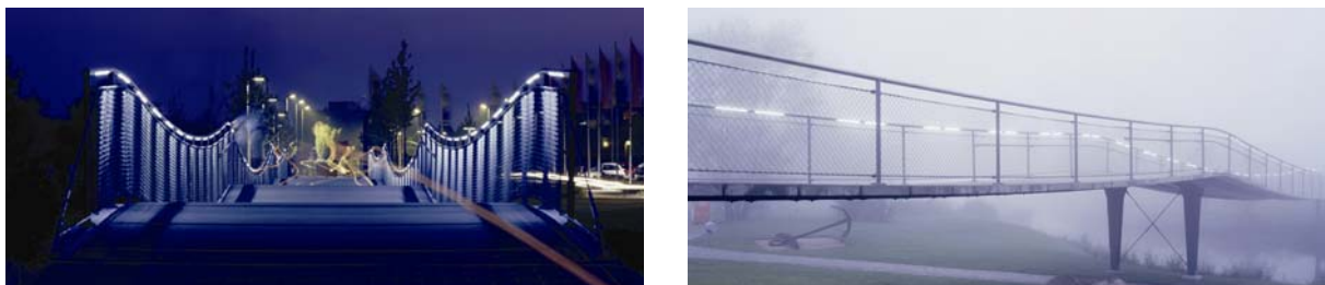
Fig.8.3 Handrail lighting at the Nordbrücke in Rostock, Germany, Engineer: Schlaich Bergemann and Partner, Architect: WES & Partner
