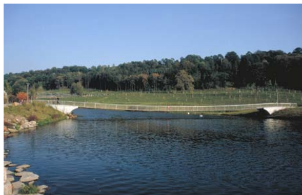
Fig. I.5 Enz Footbridge; State Garden Show in Pforzheim, Germany (1992), Engineers: Schlaich Bergermann and Partner, Architects: Knoll, Reich, Lutz
