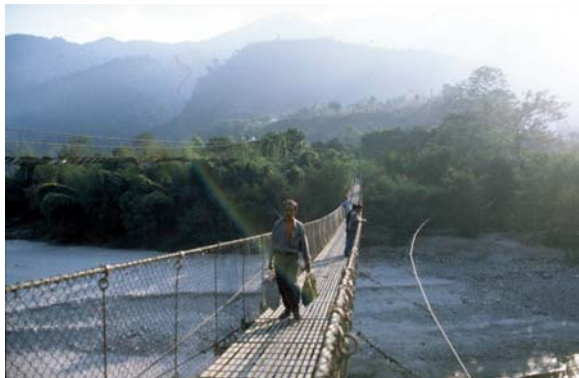
Fig. 5.21 Footbridge in Nepal with lateral cables
