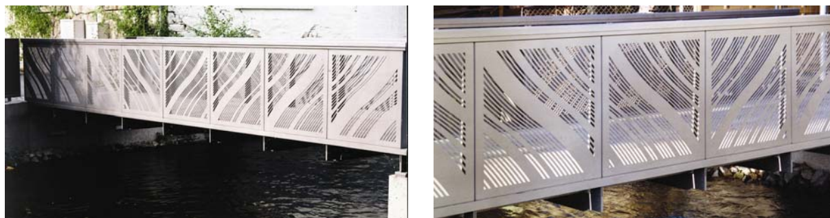
Fig. 7.4 Katherinenbrücke, Grossenhain, Germany, Engineer: ifb frohloff staffa kühl ecker, Architect: Martin Sauerzapfe Architekten [91]
