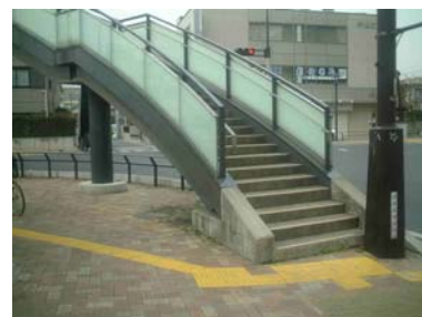
Fig. 2.3 Entrance and remaining width on sidewalk
