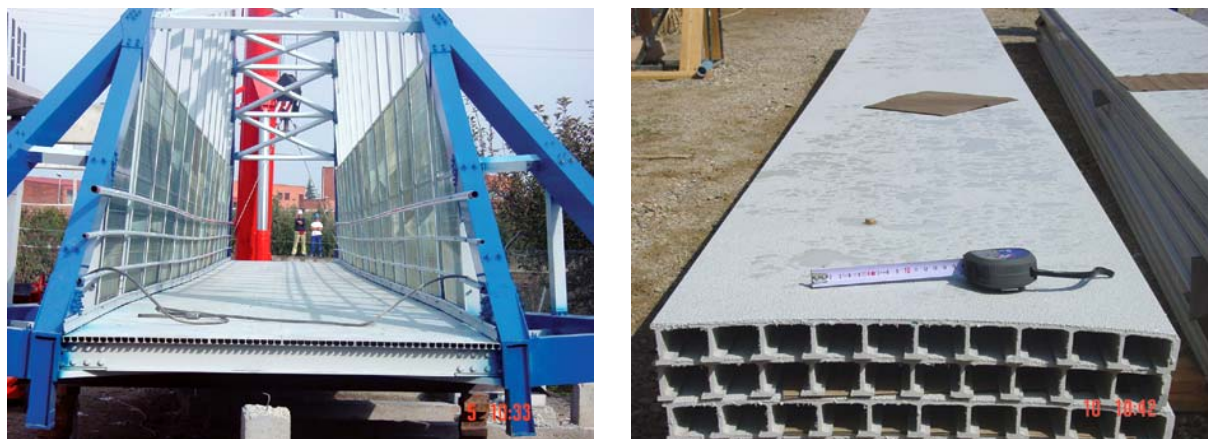
Fig. 6.5 FRP surfacing, Bridge in Lleida, Spain, Engineer: M. Dolores G. Pulido, Juan A. Sobrino
