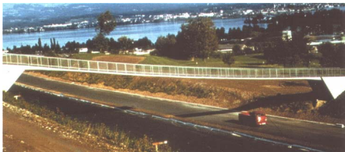
Fig. I.4 Bicherweid Footbridge, Switzerland, designed by R. Walther.
