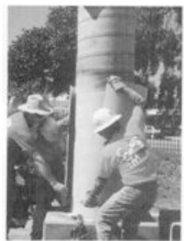
Fig. 9: Examples of prefab shapes for strengthening. (a) Angle, (b) application of angles, (c) shell.
