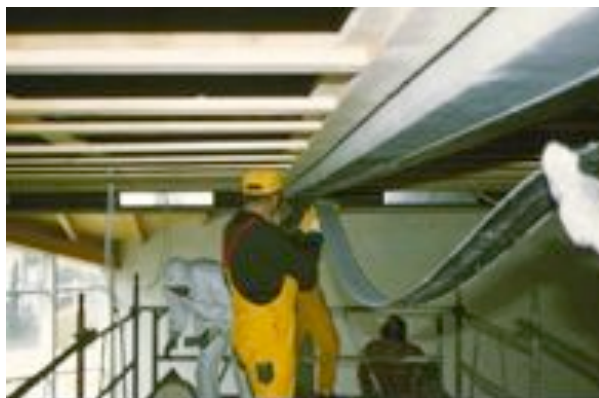
Fig. 15: Flexural strengthening of RC beam with CFRP strips.
