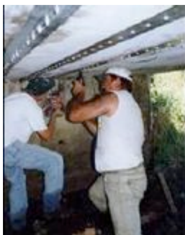
Fig. 12: (a) Mechanically-fastened FRP. (b) Detail of end anchorage with a combination of anchors and powder actuated nails.
