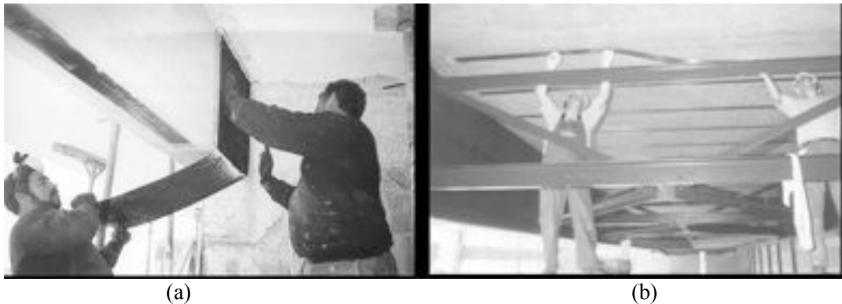
Fig. 3: (a) Hand lay-up of CFRP sheets or fabrics. (b) Application of prefabricated strips.
