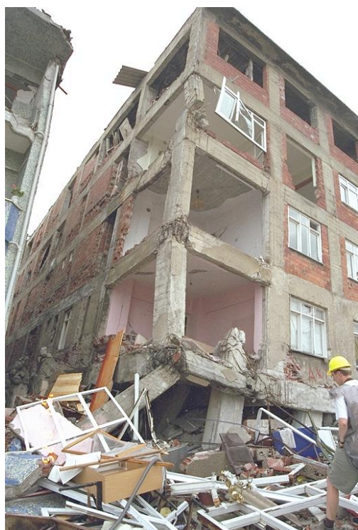
a) Building overview
