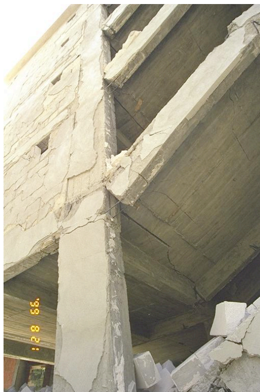
Fig. 2: Damage to non-ductile RC beam during 1999 Kocaeli earthquake [Sezen et al., 2000]
