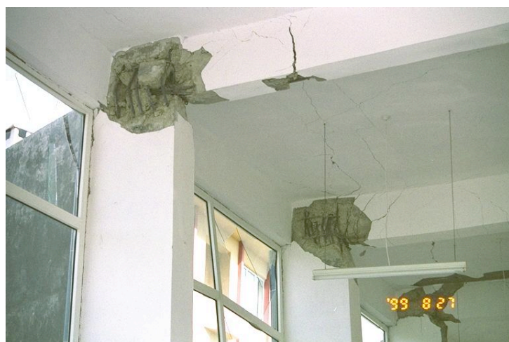
Fig. 4: Damage to a new RC moment-frame beam-column joints in 1999 Kocaeli earthquake [Sezen et al., 2000]
