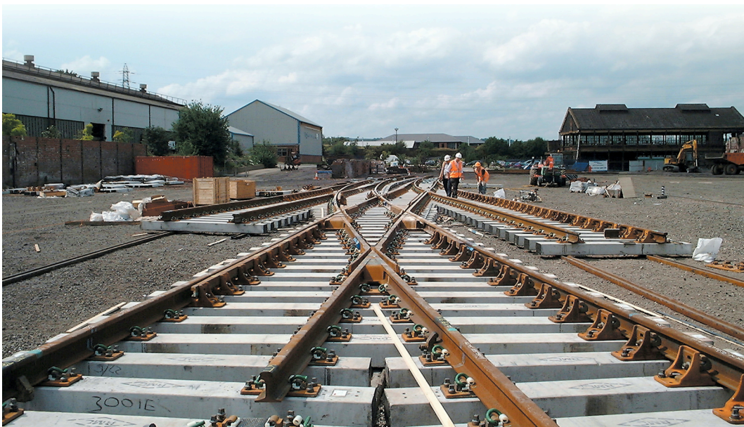
Figure 2-3: Trial assembly of crossover before installation, Balfour Beatty Rail Products, Sandiacre, UK (2004)
