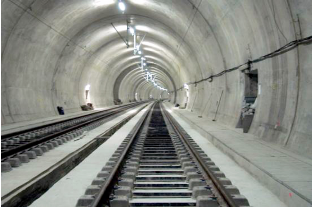
Figure 2-4: Slab track in tunnel, Réseau Ferre de France, Marseille tunnel high speed line (2003)
