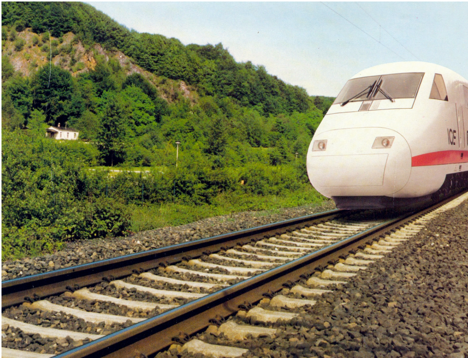
Figure 7-2: Track in Germany with Vossloh rail fastenings (2002)
