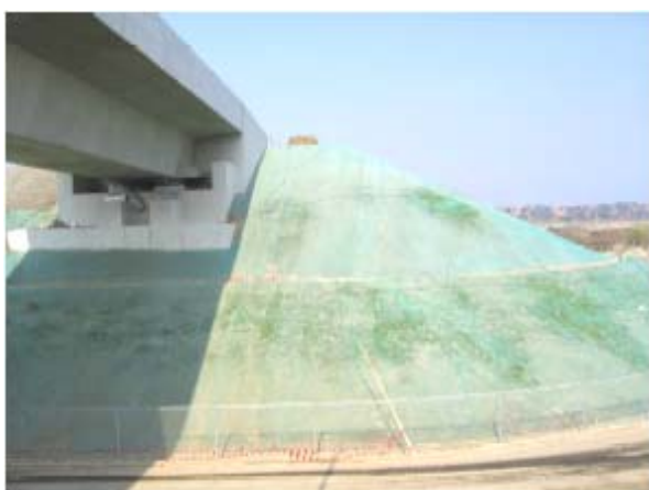
Fig. 8-15: Abutment with extended seating length and special bearings (Figures available electronically on fib website; see production note on p. ii)
