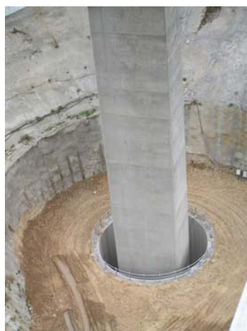
Fig. 4-12: Use of a 'pre-shaft' to increase the pier length in an Egnatia bridge (Metsovitikos) (Figure available electronically on fib website; see production note on p. ii)
