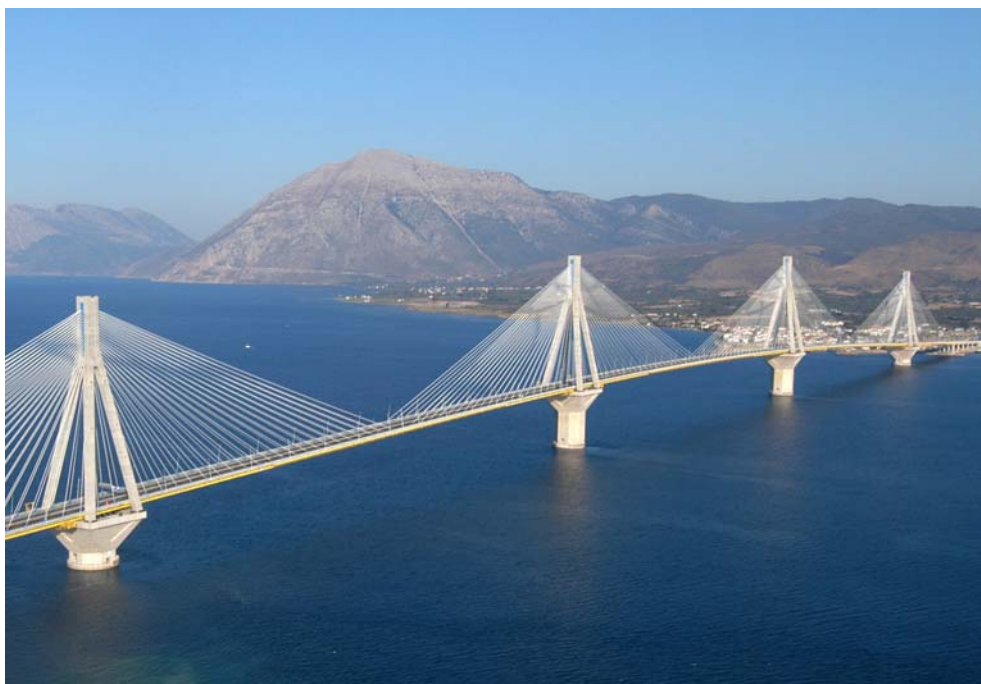
Fig. 8-19: Rion Antirion bridge (Figure available electronically on fib website; see production note on p. ii)
