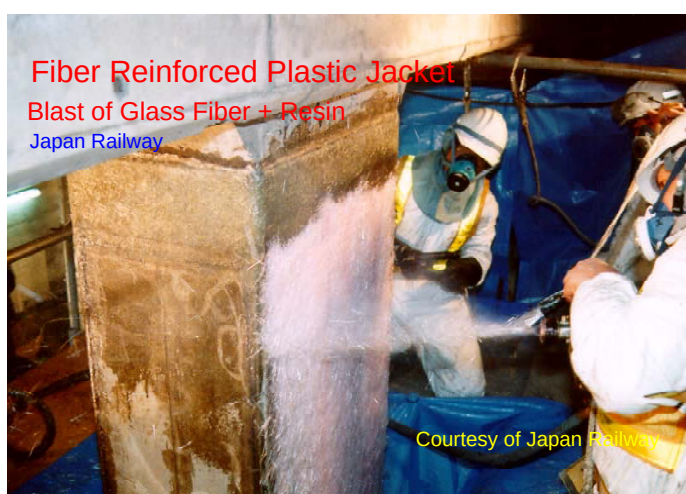
Fig. 11-34: Glass fiber jacketing (courtesy of JR Research Institute) (Figure available electronically on fib website; see production note on p. ii)
