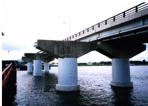
Fig. 11-31: Piers retrofitted by aramid fiber sheet [Kato et al. (2001)] (Figure available electronically on fib website; see production note on p. ii)
