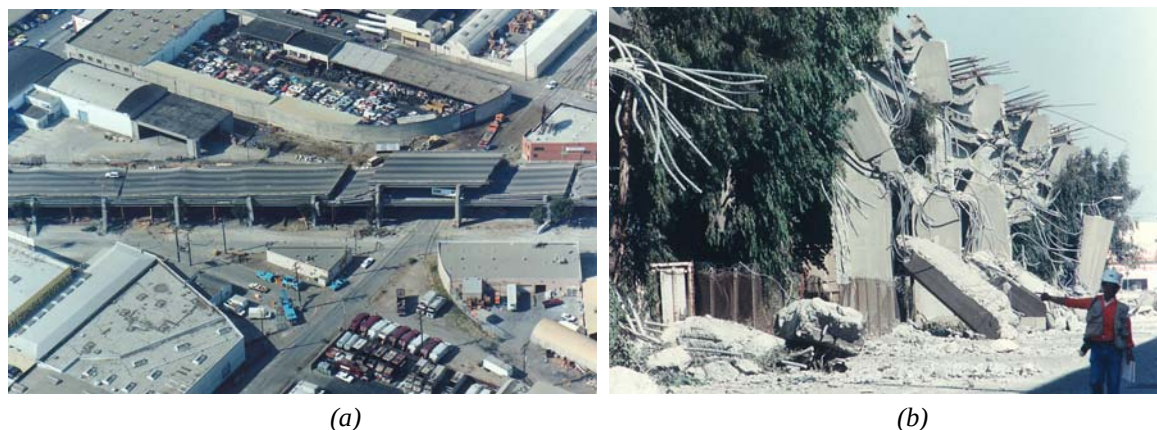
Fig. 11-43: Collapse of Cypress viaduct (Courtesy of Caltrans) (Figure available electronically on fib website; see production note on p. ii)
