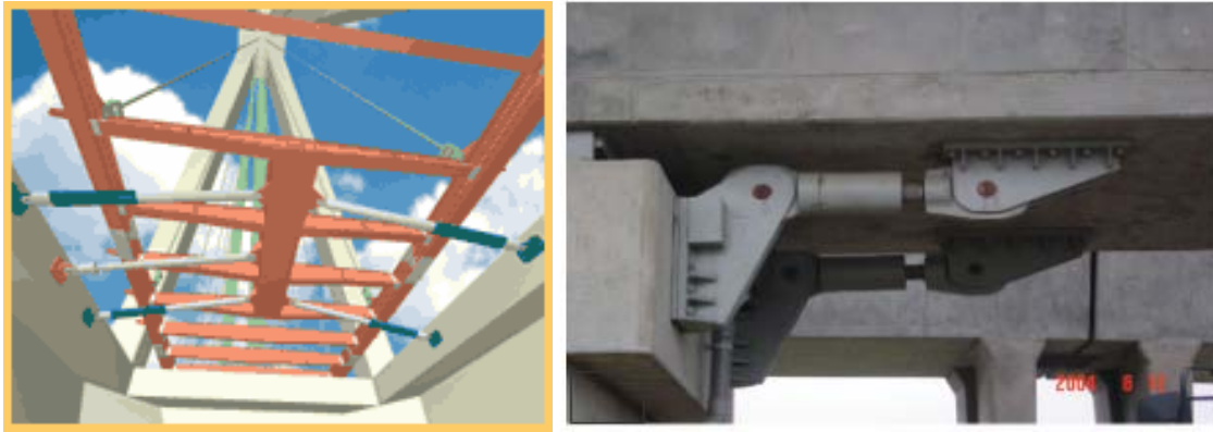
Fig. 6- 25: Representation of the viscous damper units in the Rion-Antirion bridge ( http://www.gefyra.gr ) (left), example of viscous dampers application to a bridge located at Yen-Chou in Taiwan (Hwang and Tseng, 2005) (right). (Figure available electronically on fib website; see production note on p. ii)
