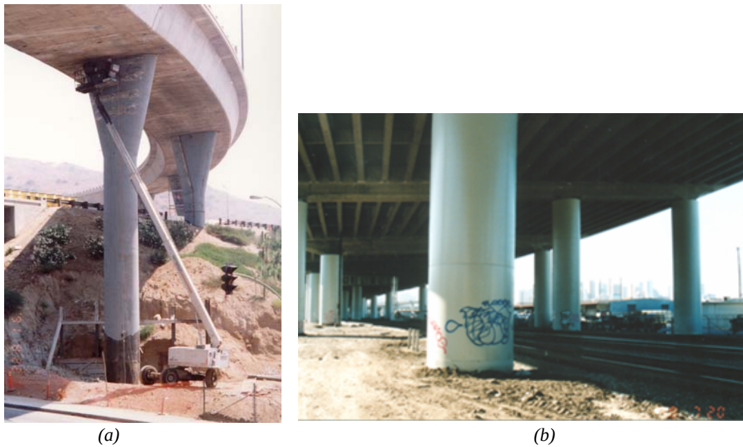
Fig. 11.2: Steel jacket retrofit of columns: (a) Los Angeles, and (b) San Francisco (Figure available electronically on fib website; see production note on p. ii)
