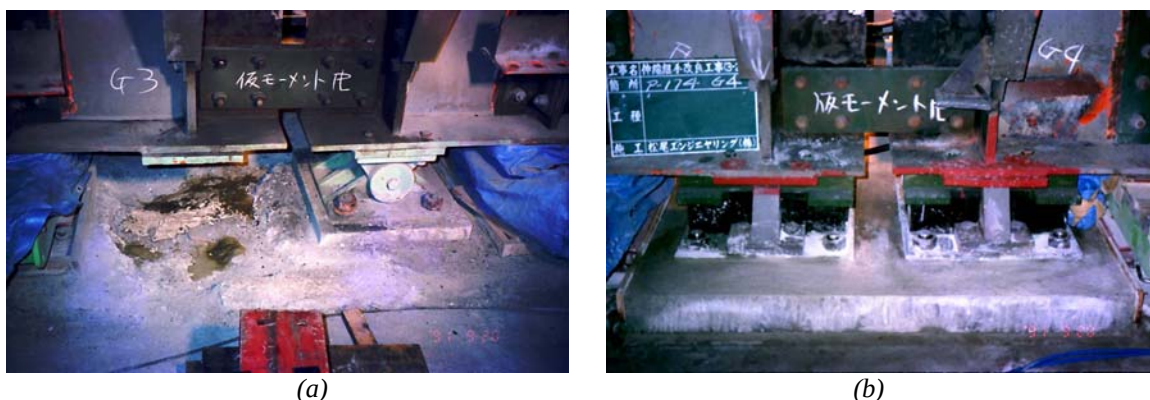
Fig. 11-68: Connection of decks and retrofit: (a) removal of existing steel bearings, and (b) set of new lead rubber bearing (courtesy of Hanshin Expressway Public Corporation) (Figure available electronically on fib website; see production note on p. ii)
