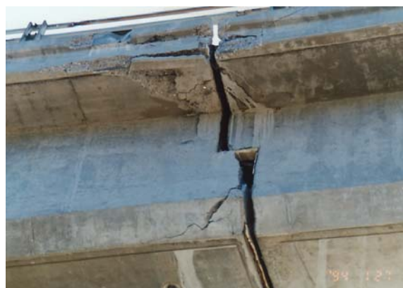
Fig. 11-61: Damage of intermediate joint due to pounding (1994 Northridge earthquake) (Figure available electronically on fib website; see production note on p. ii)
