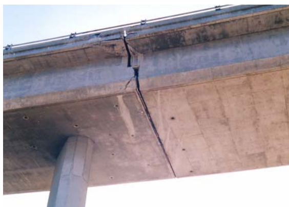
Fig. 11-61: Damage of intermediate joint due to pounding (1994 Northridge earthquake) (Figure available electronically on fib website; see production note on p. ii)
