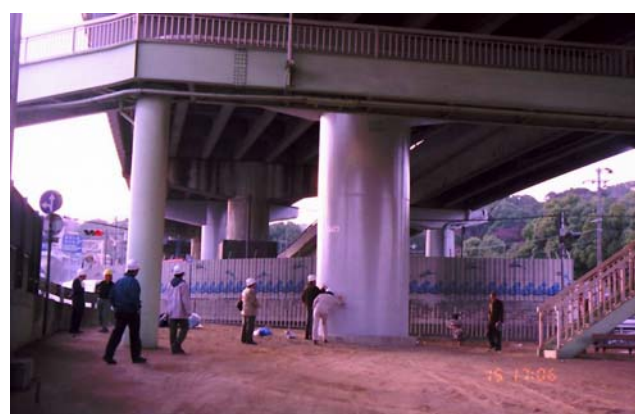
Fig. 11-4: Steel jacket retrofit at Hanshin Expressway in 1989, which was effective during the 1995 Kobe earthquake
