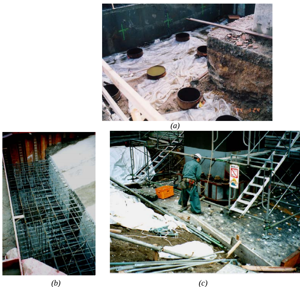
Fig. 11-52: Footing retrofit: (a) extension of footing and new piles (California, USA), (b) extension of footing and new piles (Japan), and (c) Overlay of footing (Japan) (Figure available electronically on fib website; see production note on p. ii)
