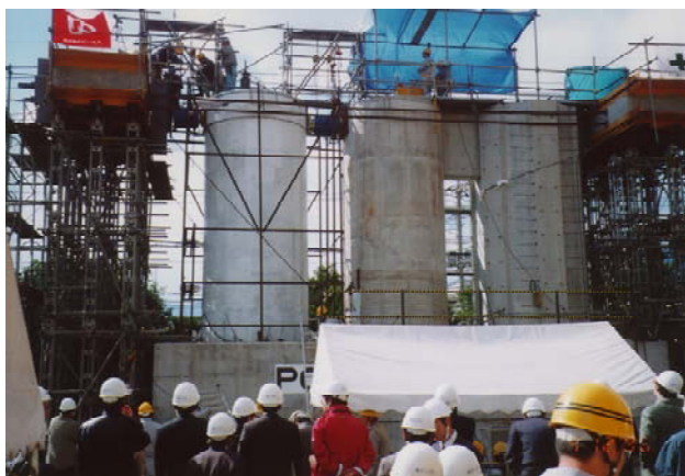
Fig. 11-36: On-site loading test on the effectiveness of PC segment jacketing (Figure available electronically on fib website; see production note on p. ii)
