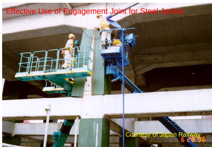
Fig. 11-14: Effective use of engagement joint for retrofit at a railway viaduct (JR Research Institute) (Figure available electronically on fib website; see production note on p. ii)
