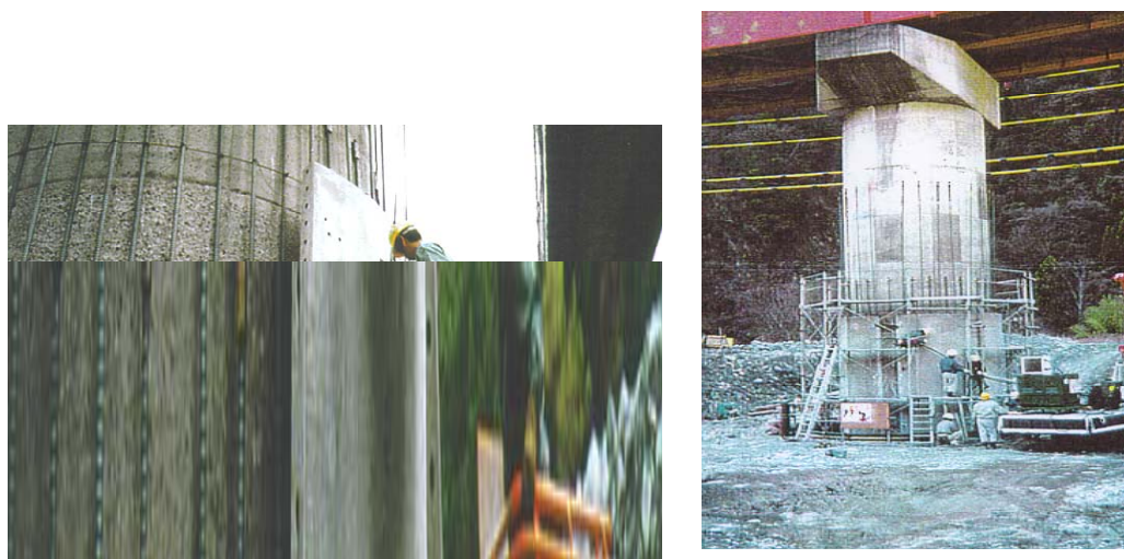
Fig. 11-35: Precast concrete segment jacket [courtesy of PS Concrete] (Figure available electronically on fib website; see production note on p. ii)
