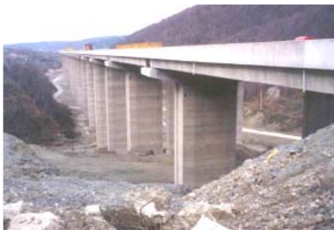
Fig. 8-5: Bolu Viaduct - view from abutment S2
