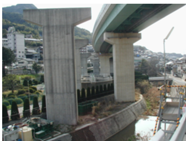
(a) before retrofit
