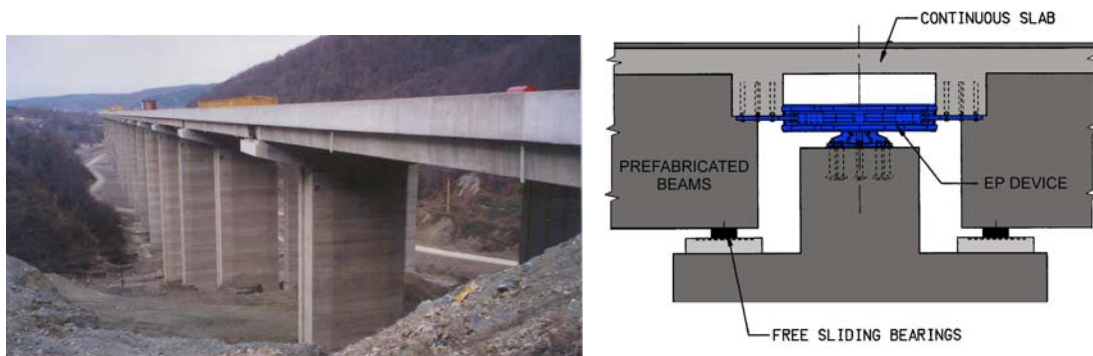
Fig. 6- 19: View of the Bolu Viaduct (Priestley and Calvi, 2003) (left) and detail of the pier top (Marioni, ALGA S.p.A.) (right). (Figure available electronically on fib website; see production note on p. ii)
