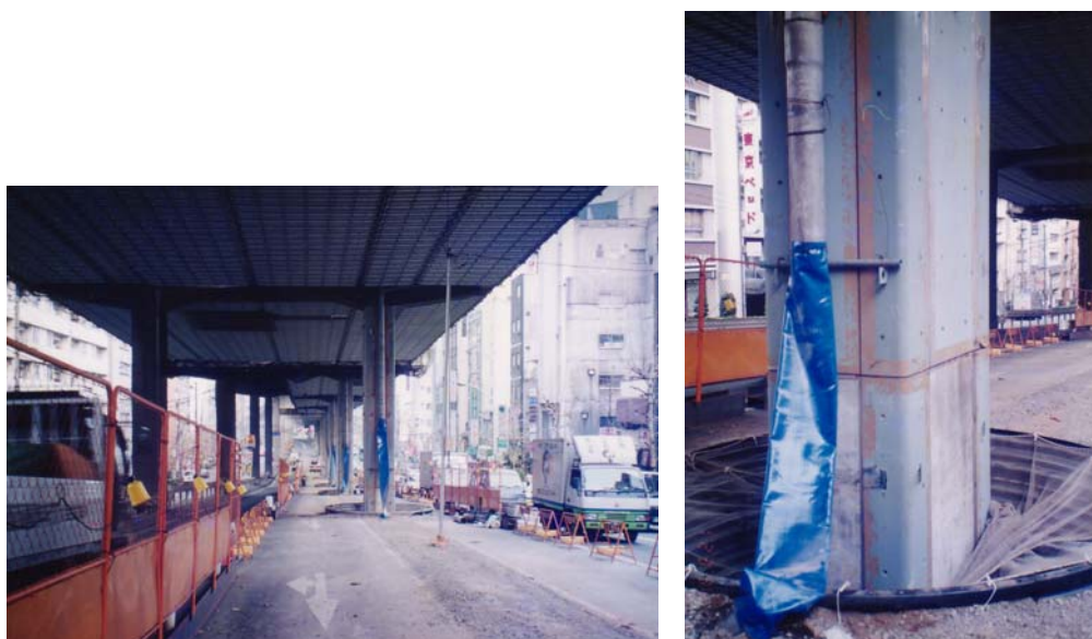
Fig. 11-12: Steel jacket retrofit for frame piers, Metropolitan Expressway, Japan (Figure available electronically on fib website; see production note on p. ii)
