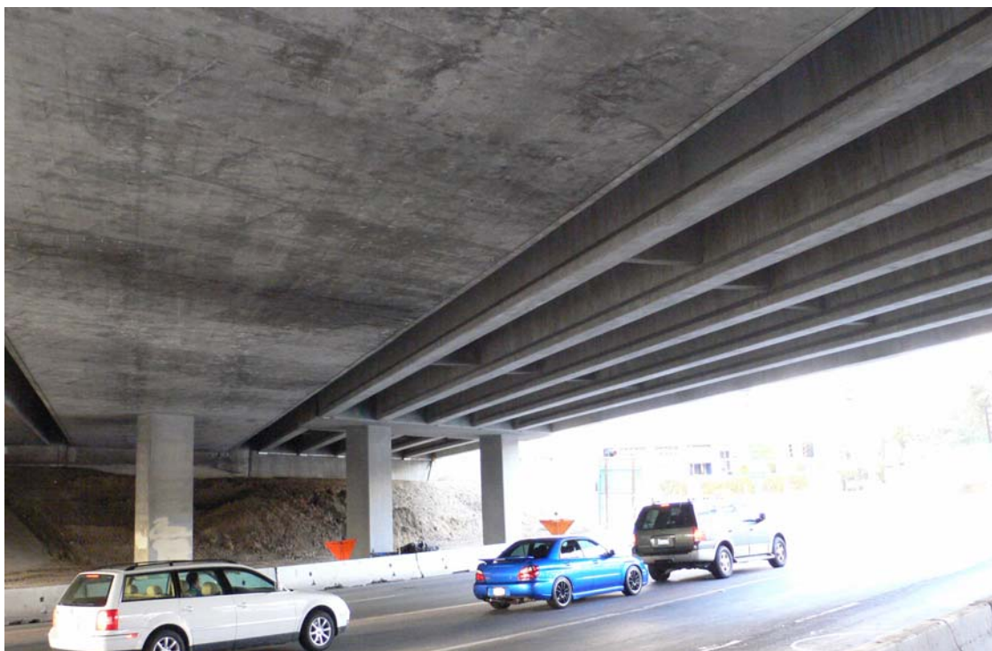
Fig. 4-10: Example of use of the use of precast I-girders on a highway bridge widening project in California (Courtesy of J. Restrepo) (Figure available electronically on fib website; see production note on p. ii)
