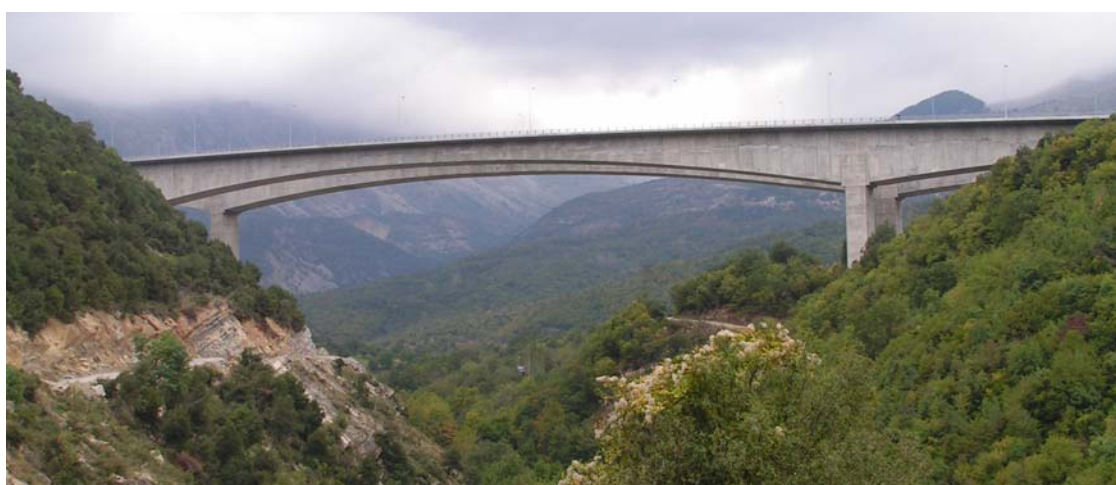
Fig. 4-2: The Votonosi Bridge near Metsovo (NW Greece); the superstructure consists of a post-tensioned single cell box girder (common in modern bridges), and its 230m central span, is the longest span so far in balanced cantilever construction in Greece (Courtesy of A. Kappos). (Figure available electronically on fib website; see production note on p. ii)
