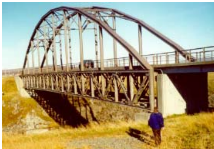
Fig. 6- 5: The Thjorsa bridge in the South Iceland Lowlands (mceer.buffalo.edu). (Figure available electronically on fib website; see production note on p. ii)
