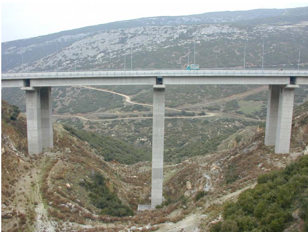
Fig. 4-7: The G2 bridge near Kavala (NE Greece); the superstructure consists of precast post-tensioned beams connected through a cast in situ top slab (typical of older construction) (Courtesy of A. Kappos). (Figure available electronically on fib website; see production note on p. ii)
