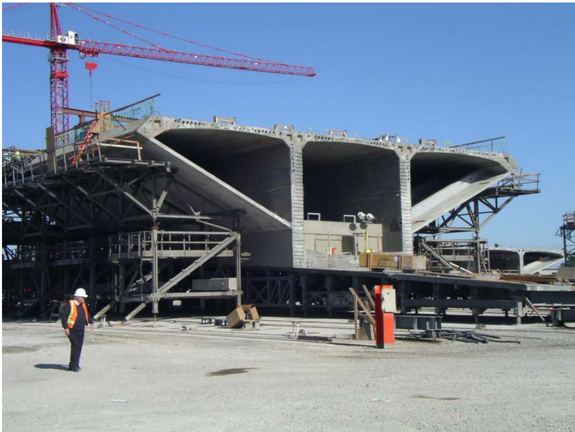
Fig. 4-9: Precast segmental elements for the construction of the San Francisco-Oakland Bay Bridge Skyway Structure (Courtesy of F. Seible) (Figure available electronically on fib website; see production note on p. ii)
