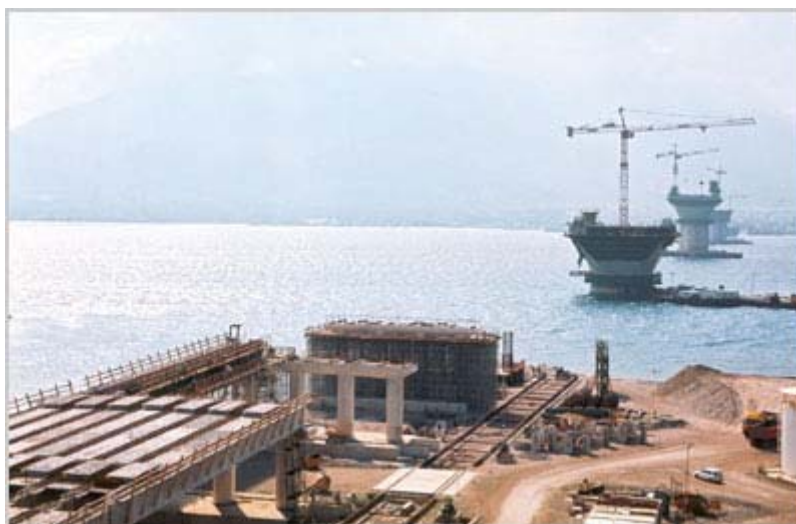
Fig.5-16: View of the Antirion access viaduct during construction (see pile cap above ground surface) (Figure available electronically on fib website; see production note on p. ii)
