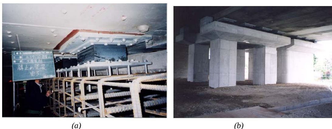
Fig. 11-67: Seismic retrofit using isolation: (a) installation of lead rubber bearings and sliding bearings, and (b) after retrofit (courtesy of Japan Highway Public Corporation) (Figure available electronically on fib website; see production note on p. ii)
