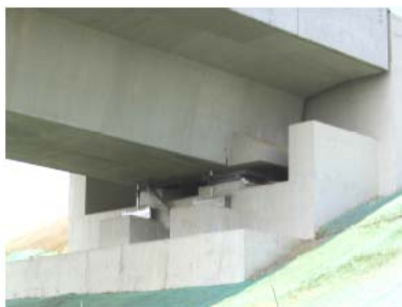
Fig. 8-15: Abutment with extended seating length and special bearings (Figures available electronically on fib website; see production note on p. ii)
