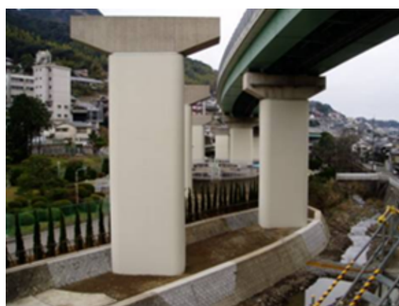
(b) after retrofit
