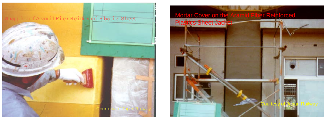
Fig. 11-30: Aramid fiber reinforced plastics jacketing for a railway viaduct [courtesy of JR Research Institute] (Figure available electronically on fib website; see production note on p. ii)
