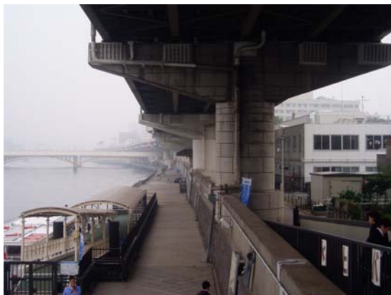
Fig. 11-3: Steel jacket retrofit at Metropolitan Expressway
