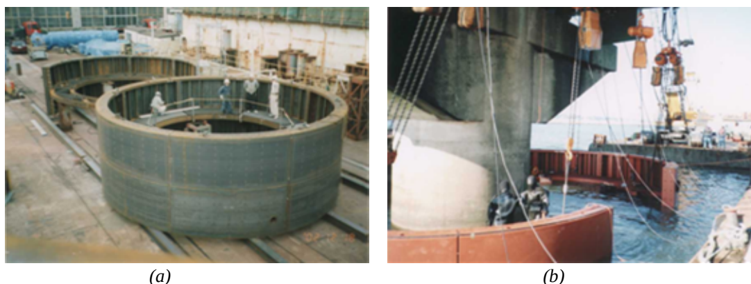
Fig. 11-55: Implementation of steel segment dry-up method: (a) assembling test, and (b) assembling the segments around the foundation [courtesy of Obayashi Construction] (Figure available electronically on fib website; see production note on p. ii)
