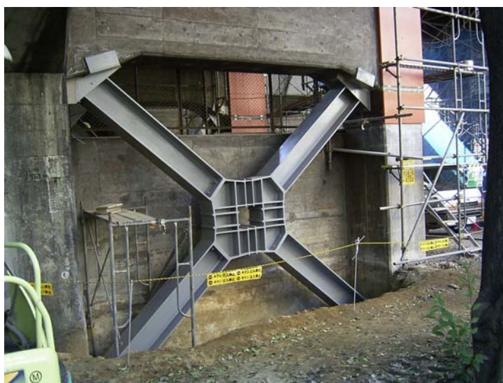
Fig. 11-73 Viaduct retrofitted using compression brace damper [Yoshida et al. (2005)] (Figure available electronically on fib website; see production note on p. ii)
