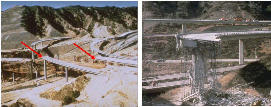
Figure 10-1: Span collapses at the Golden State-Antelope Valley interchange collectors during the 1971 San Fernando (left) and the 1994 Northridge (right) earthquakes (courtesy of USGS). (Figure available electronically on fib website; see production note on p. ii)
