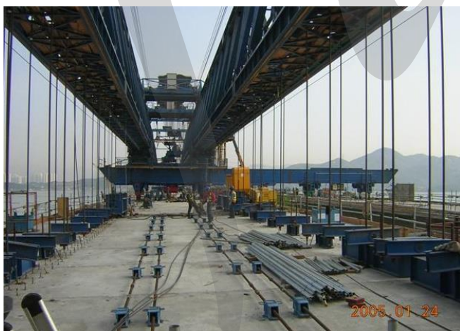
Figure 5-48: Temporary post tension suspension system for overhead girder
