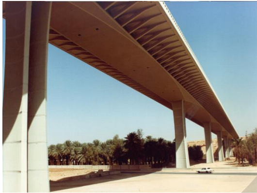
Figure 4-23: Examples of twin leaf piers continuous with the deck. The use of taper and curvature and connection between the leaves allows pier stiffness to be varied [Srinivasan, 2004]
