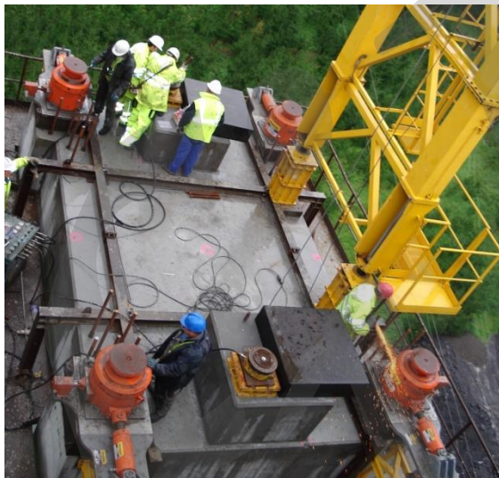
Figure 4-10: Pier head with balanced cantilever method
