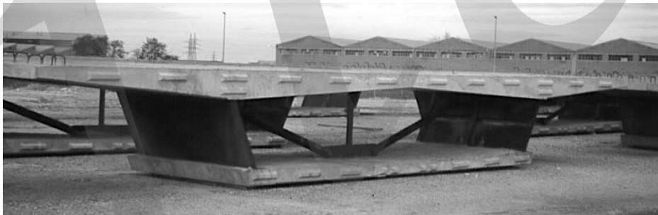
Figure 4-9: Segment with webs in steel
