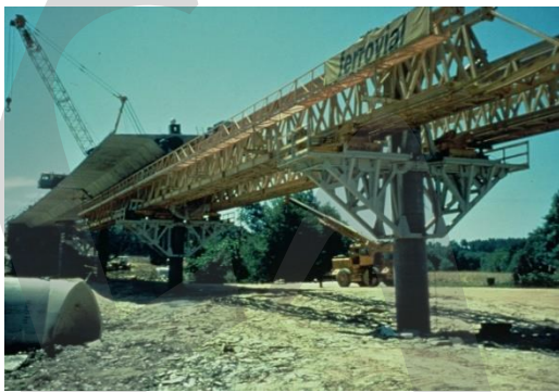
Figure 3-6: Underslung truss (Miño viaduct)
