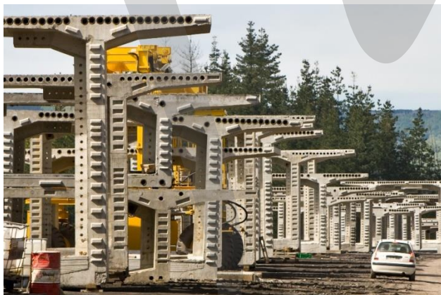
Figure 5-3: Example of joint with multiple shear keys
