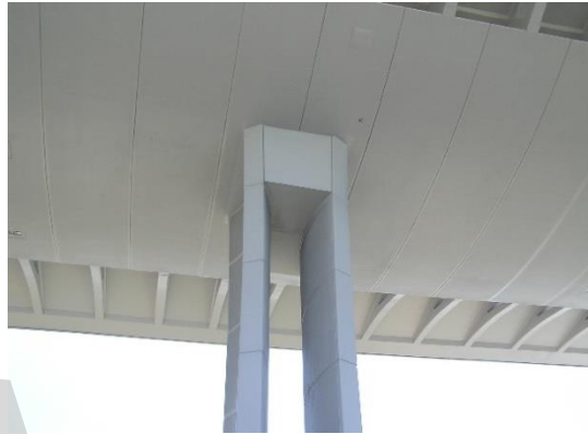
Figure 4-23: Examples of twin leaf piers continuous with the deck. The use of taper and curvature and connection between the leaves allows pier stiffness to be varied [Srinivasan, 2004]
