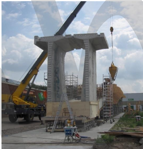
Figure 5-25: Initial segment and bottom slab cast in long-line
