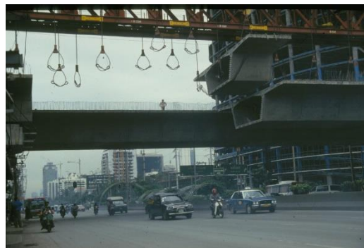
Figure 4: Assembling of segments
