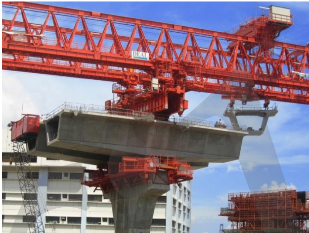
Figure 5-82: Erection by balanced cantilever method
