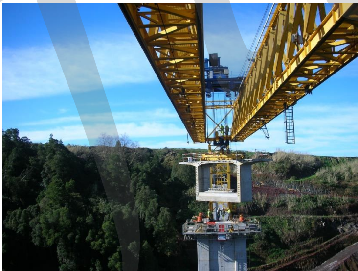
Figure 5-80: Erection of precast pier segment
