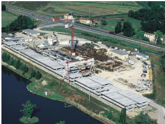
Figure 5-17: Temporary prefabrication yard
