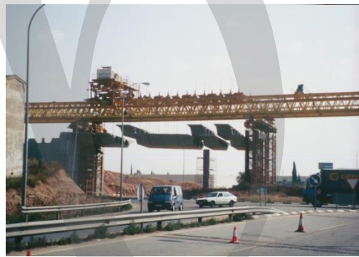
Figure 3-7: Overhead gantry (Alcalá viaduct)
