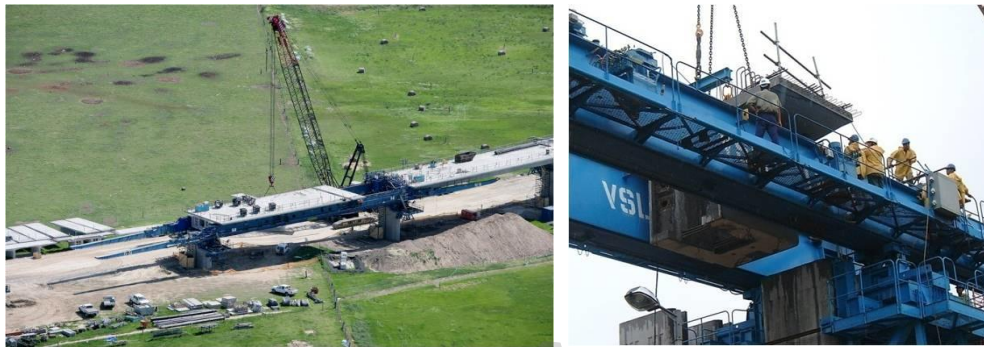
Figure 5-61: Segment loading by external crane on an underslung girder
