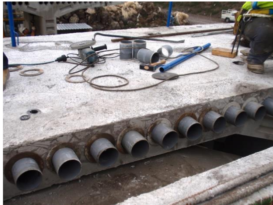
Figure 4-31: Metallic rings to leave the room for gaskets
