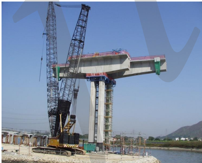
Figure 5-86: Segment erection by crane
