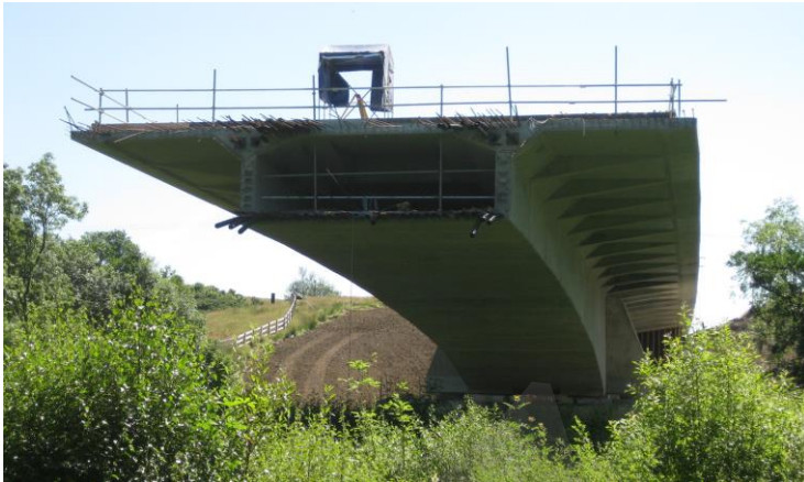
Figure 4-14: Box with ribs
