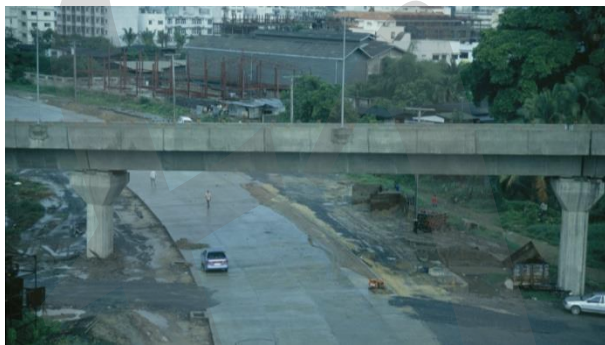
Figure 4-21: Simply supported spans with span-by-span-method
