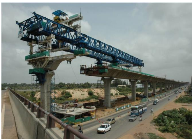
Figure 5-49: Transfer of front support during launching process
