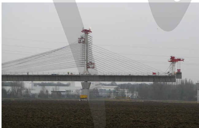
Figure 3-9: Progressive placement method: staying mast and swivel crane
