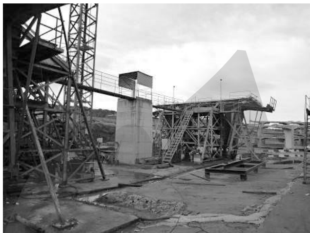
Figure 5-6: Survey base station close to precast cell
