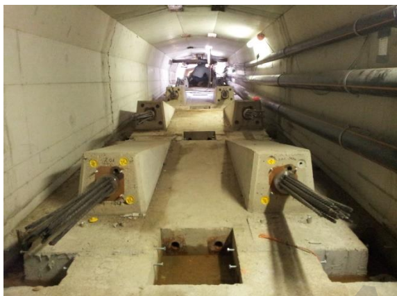
Figure 2: Tendon anchor at bottom plate
