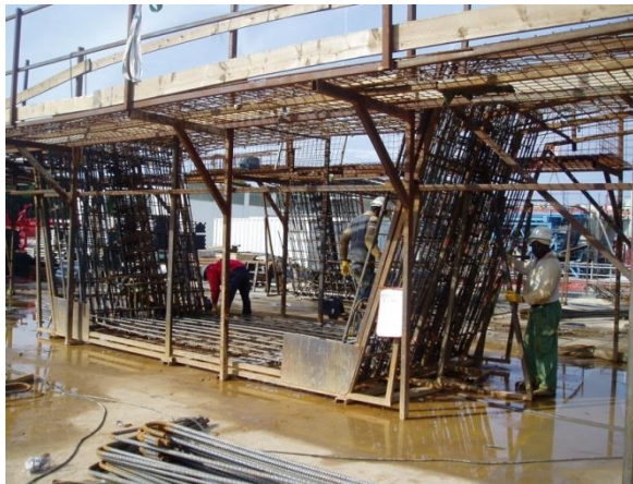
Figure 5-31: Reinforcement cage prefixed in a jig
