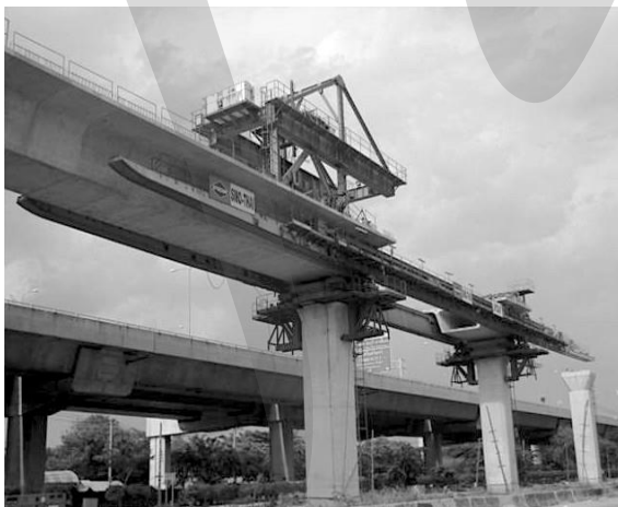
Figure 5-60: An underslung girder with its bracket system and segment loader from deck
