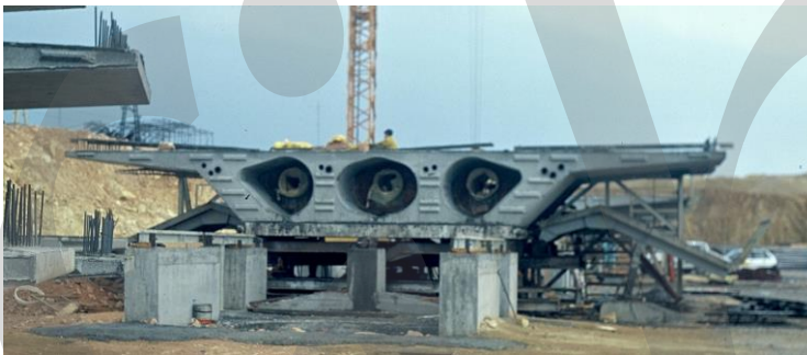
Figure 4-15: Hollowed slab with transversal cantilevers
