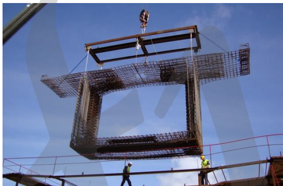
Figure 5-22: Prefixed rebar cage lifted by a crane, to be positioned in the cell
