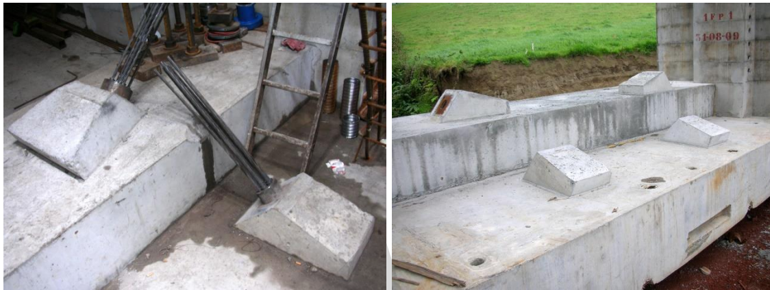
Figure 5-75: Temporary nailing to ensure the stability of both cantilevers
