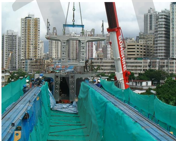
Figure 5-63: Placing segment above an underslung girder; tarpaulin used to catch excess glue and for safety over an urban area
