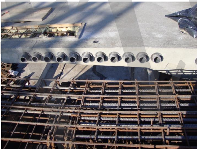
Figure 5-36: Plastic couplers and washers placed at the joint before pouring the concrete
