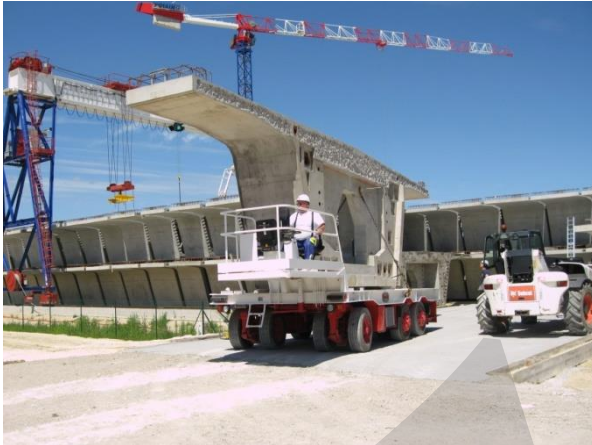
Figure 5-23: Purpose-made segment carrier
