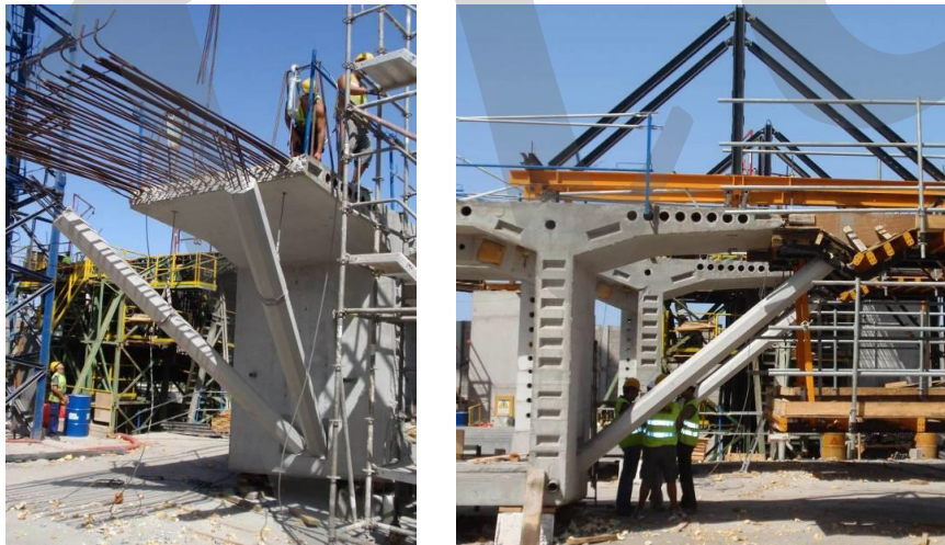
Figure 3: Preparation of the segment to complete the second phase of the precast
