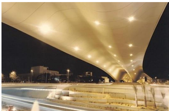
Figure 4-2: 131-m span balanced cantilever erection (Al-Khaleej viaduct, Riyadh, KSA)
