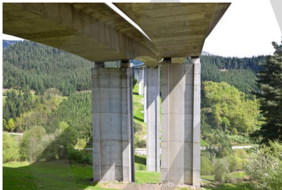
Figure 4-24: Simply supported deck over pier
