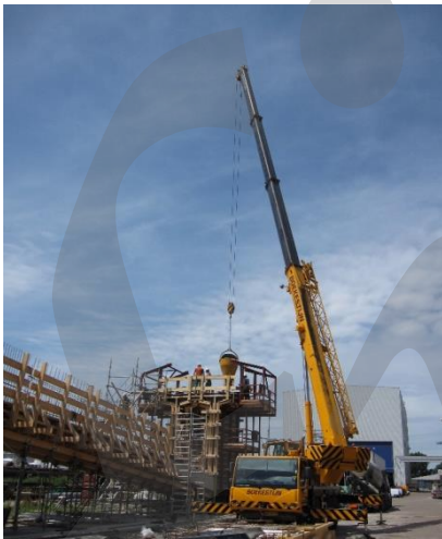
Figure 5-25: Initial segment and bottom slab cast in long-line
