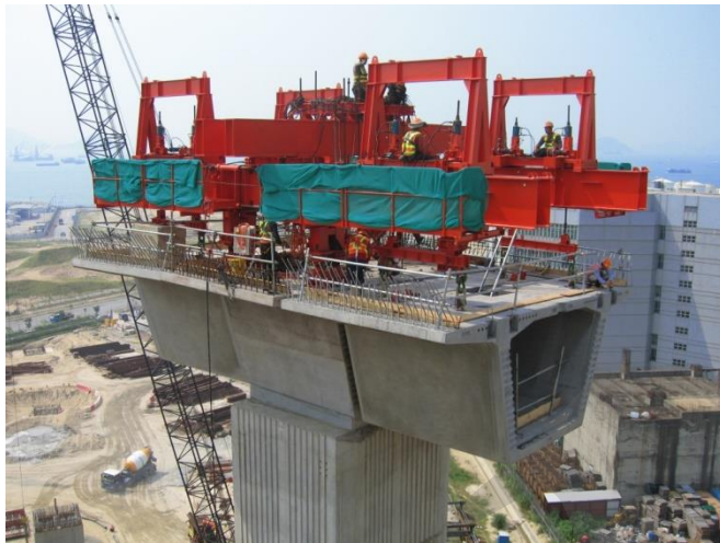
Figure 5-83: Erection of first field segment against in-situ segment on pier
