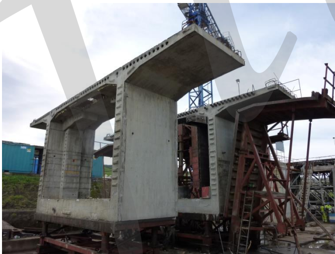
Figure 5-27: Segments cast on a short-line precast yard
