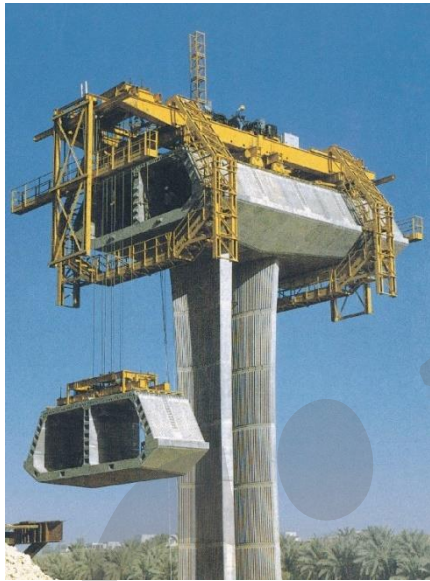
Figure 3-4: A variant of balanced cantilever erection by bespoke erection machine –integrated walkway for access around the segment for gluing (Quarashia Viaduct, KSA) [Srinivasan, 2004]
