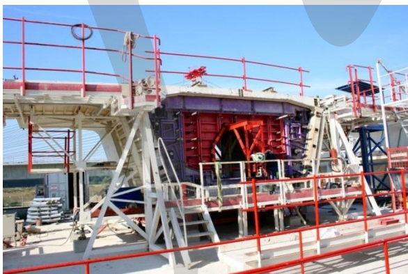
Figure 5-33: Short-line bed dedicated to pier and end segments
