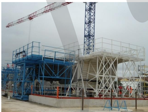
Figure 5-30: Short-line precasting bed
