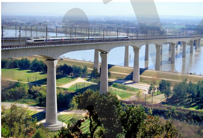
Figure 4-33: Viaducts in Avignon
