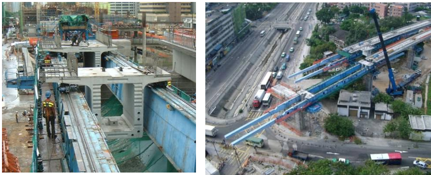
Figure 5-64: Trolley system used for segment displacement
