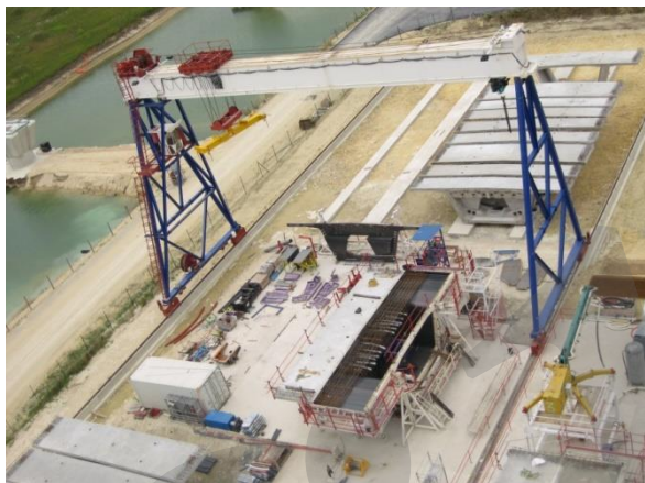
Figure 5-15: Production area with short-line bed and storage area
