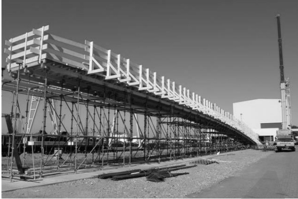
Figure 5-24: Preparation of deck bottom formwork in long-line
