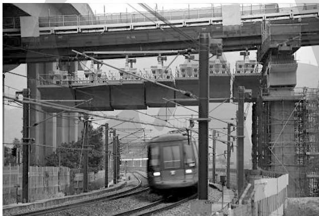
Figure 5-38: Overhead girder over live train tracks
