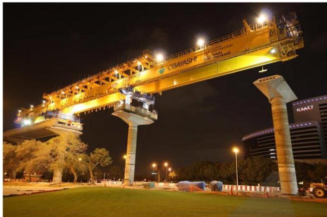
Figure 5-46: Overhead girder ready to start span erection for a U-shape precast segment
