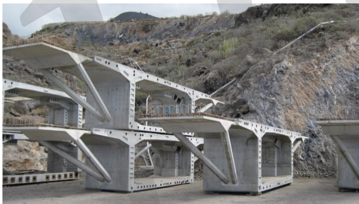
Figure 4-13: Box with struts
