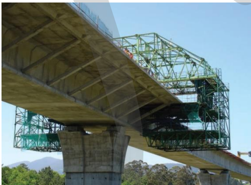
Figure 6-1: Example of segmental construction combined with transversal in-situ cantilevers
