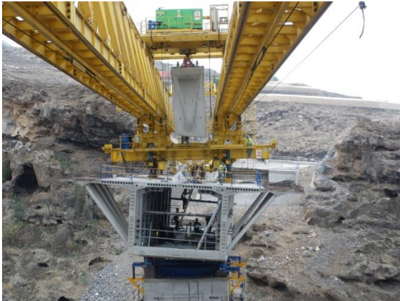
Figure 4-5: Launcher leg in transversal slope with balanced cantilever method
