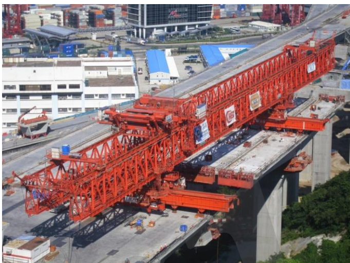
Figure 5-84: Launching girder used for the erection of the East Tsing Yi viaduct
