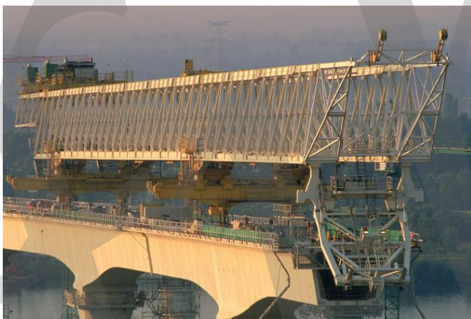
Figure 5-85: Launching girder used on the Avignon project
