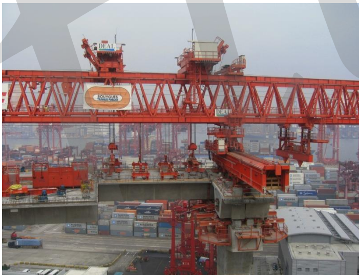
Figure 5-90: End-span hung to the launching girder
