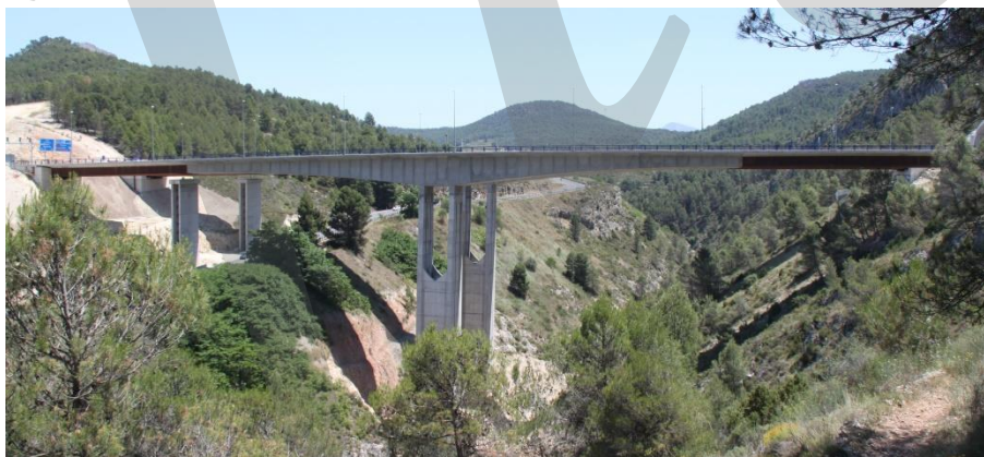
Figure 3: Bridge finished (before demolishing the provisional piers)
