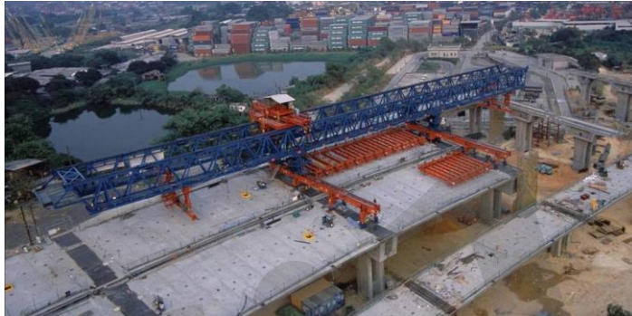
Figure 5-43: Continuous span erected as in-fill span
