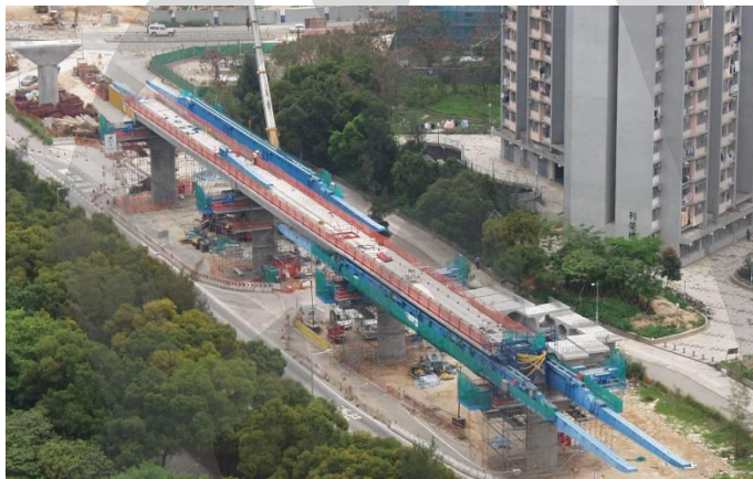
Figure 5-42: Isostatic span erected by underslung girder
