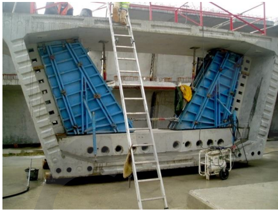
Figure 5-34: Second stage of concreting of a diaphragm wall segment
