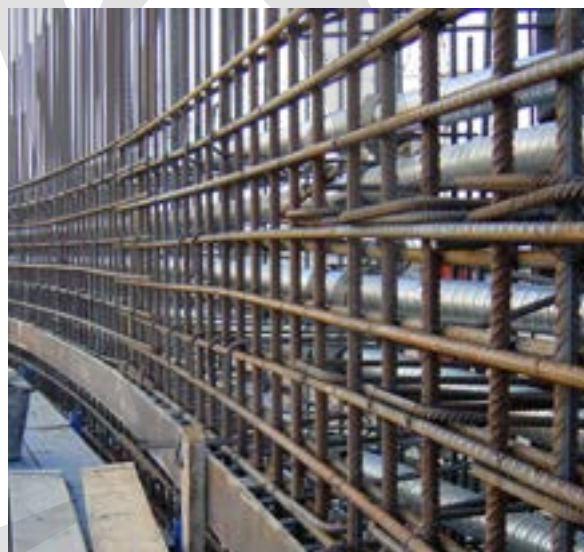
b) Installation of duct for horizontal tendons
