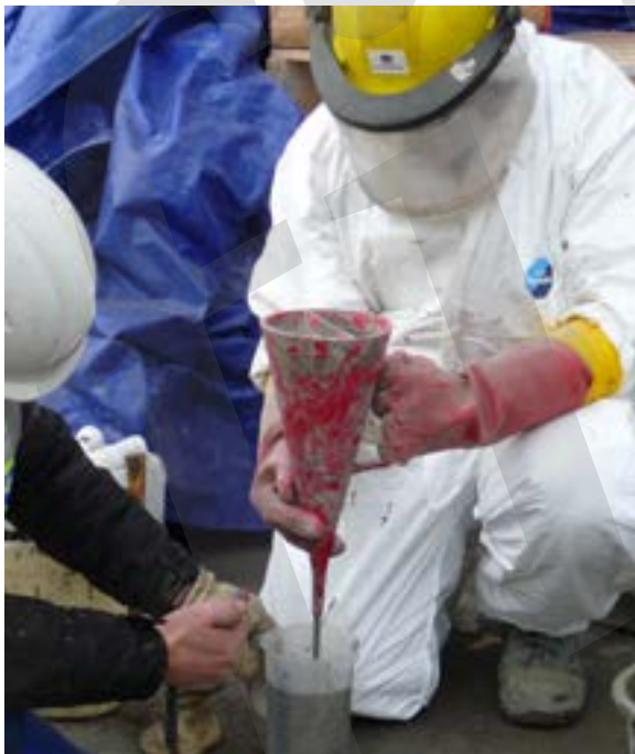
e) Testing of grout before grouting
