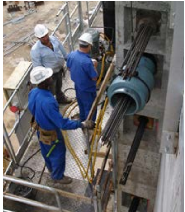
d) Stressing of horizontal tendons
