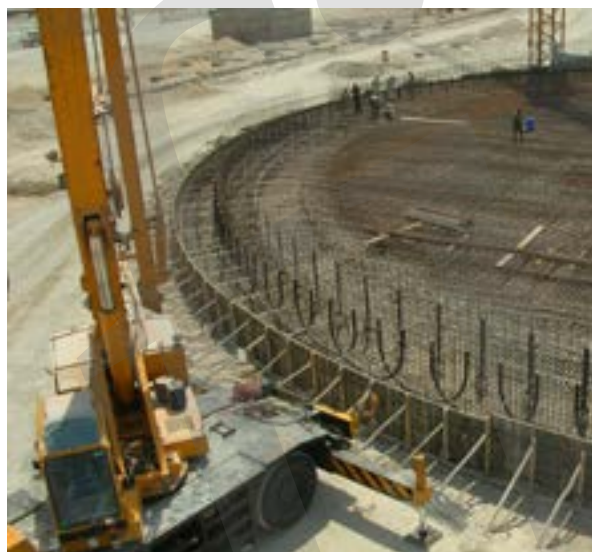
a) Installation of ducts for loop tendons
