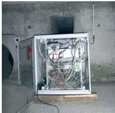
Fig. 4 Installation des Computers. Installation of computer.
