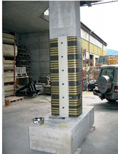
Fig. 4 Renforcement colonnes P3 et P4. Strengthening of columns P3 and P4.
