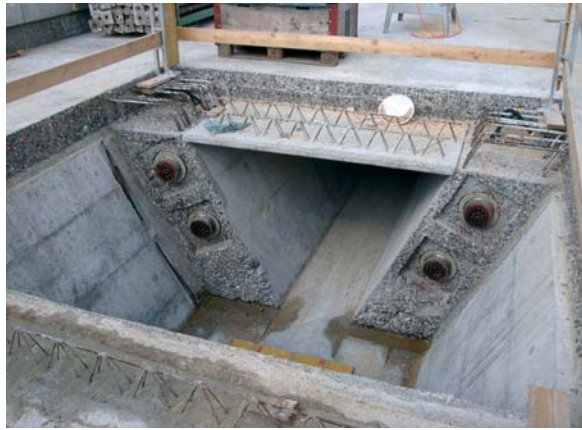
Fig. 5 Typische Abspannstelle. Typical anchoring of prestressing tendons.
