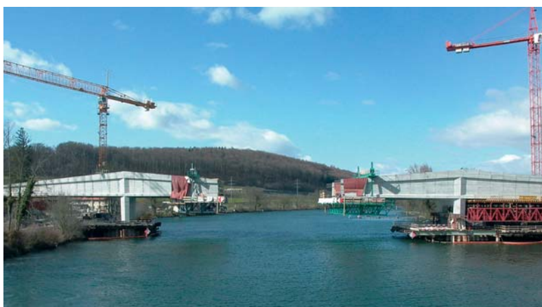
Fig. 5 Freivorbauphase. Free cantilever construction stage.
