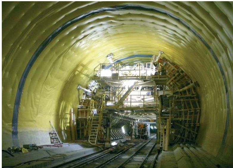
Fig. 4 Gewölbeschalwagen. Montage der Stirnschalung (© Arge Transco). Lining formwork car. Installation of the bulkhead formwork (© consortium Transco).
