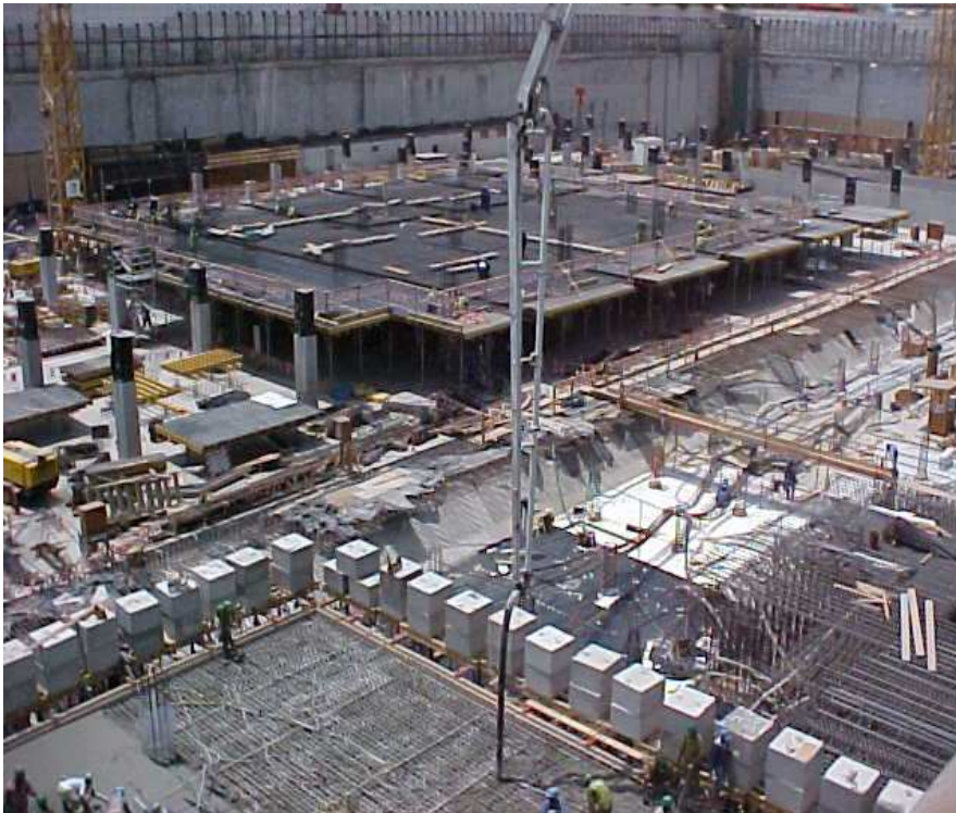
10,000 m 2 Bur-Juman Bodenplatte, Dubai
